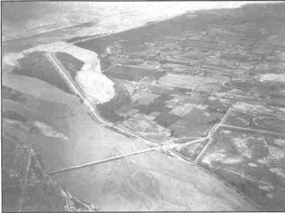
Figure 21: Central Avenue Bridge on May 26, 1930 (from Daves, 1994).
