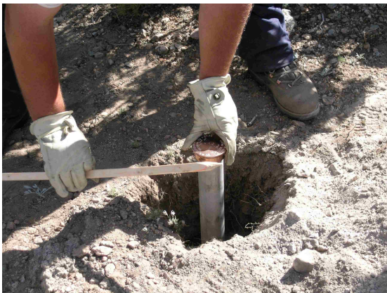
Figure 35. Setting the newly-surveyed corner brass cap.
