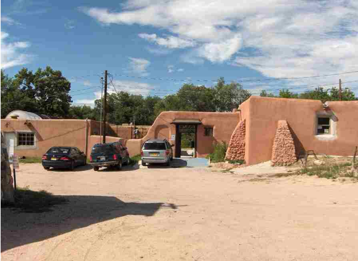
Figure 38 at the Plaza del Alcalde, a view looking north at a portion of the built environment from the plaza in front of the chapel taken in 2010 (courtesy Dr. Jose Rivera, UNM).
