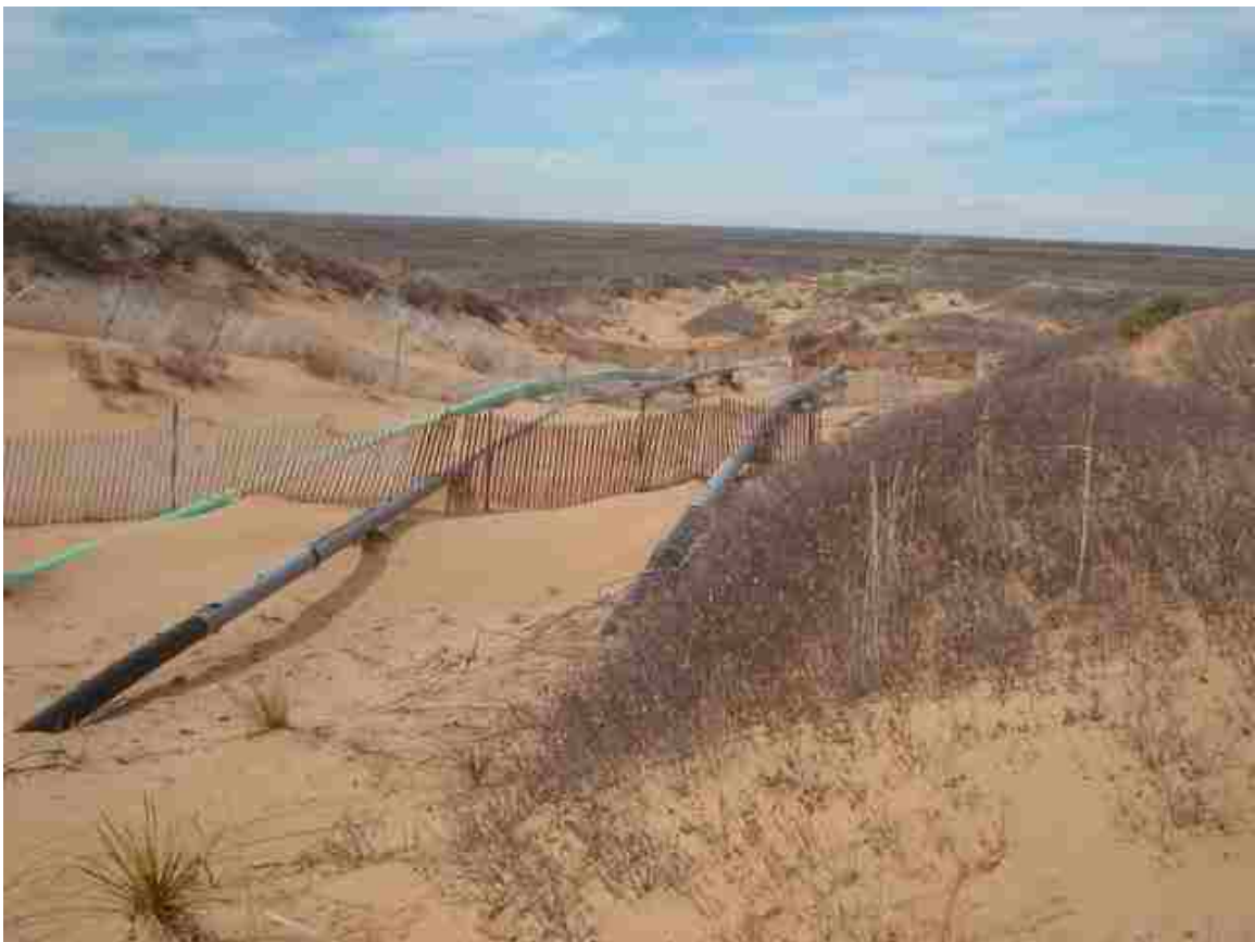
Figure 1: Pipelines Exposed by Blowout . Blowout on right of way located within the Mescalero sand sheet. Photo: Knutt Peterson
