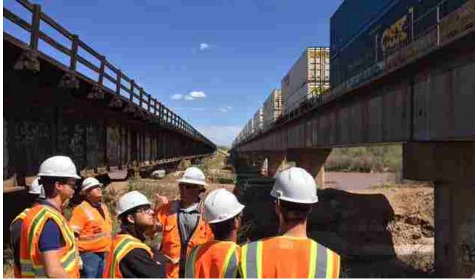
Figure 2-1. Visual inspection of railroad bridges.
