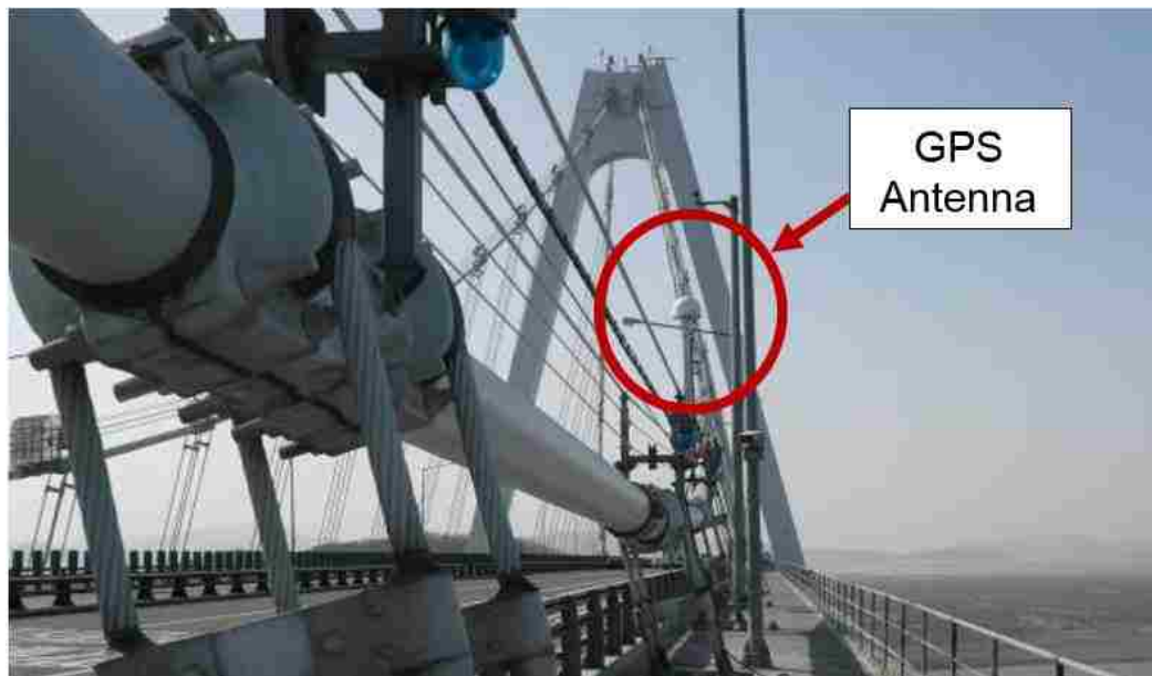
Figure 2-4. GPS for bridge displacement measurement (Carnenbroeck 2015)
