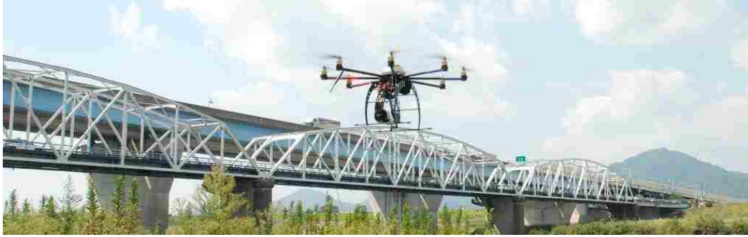
Figure 2-9. UAS for bridge monitoring (Smart Sensys 2017)
