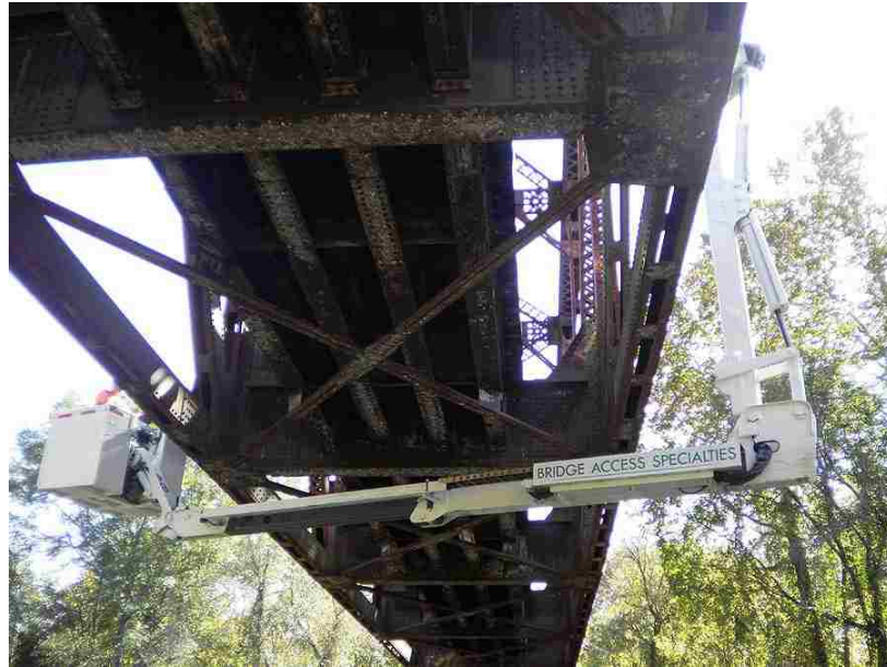
Figure 1-2. Inspectors monitoring a railway bridge (Bridge access specialties 2017)
