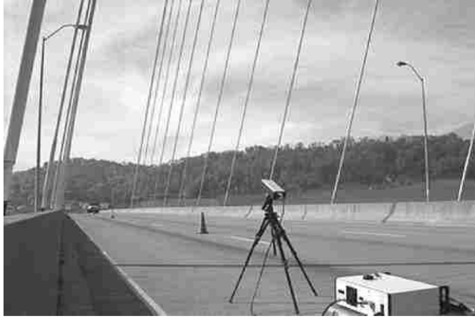
Figure 2-8. Laser doppler vibrometer for structural health monitoring of a highway bridge (Mehrabi, 2006)
