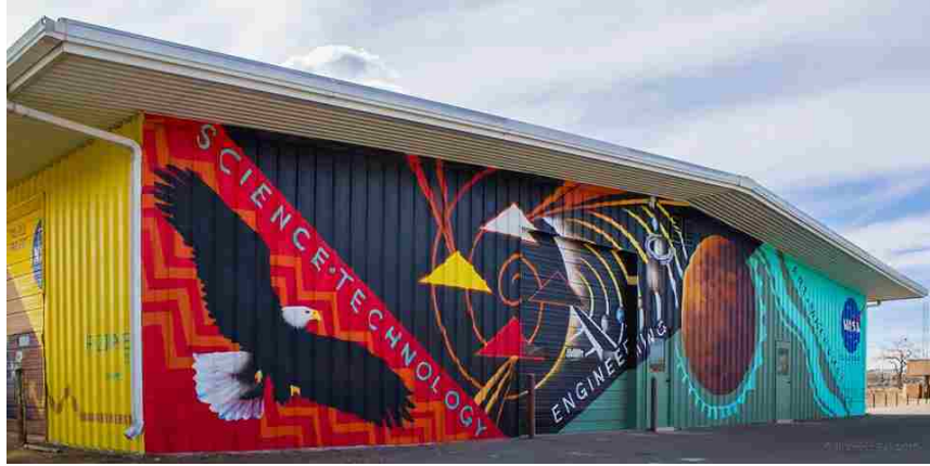
Figure 4.2: Main Mars Yard Exterior East
