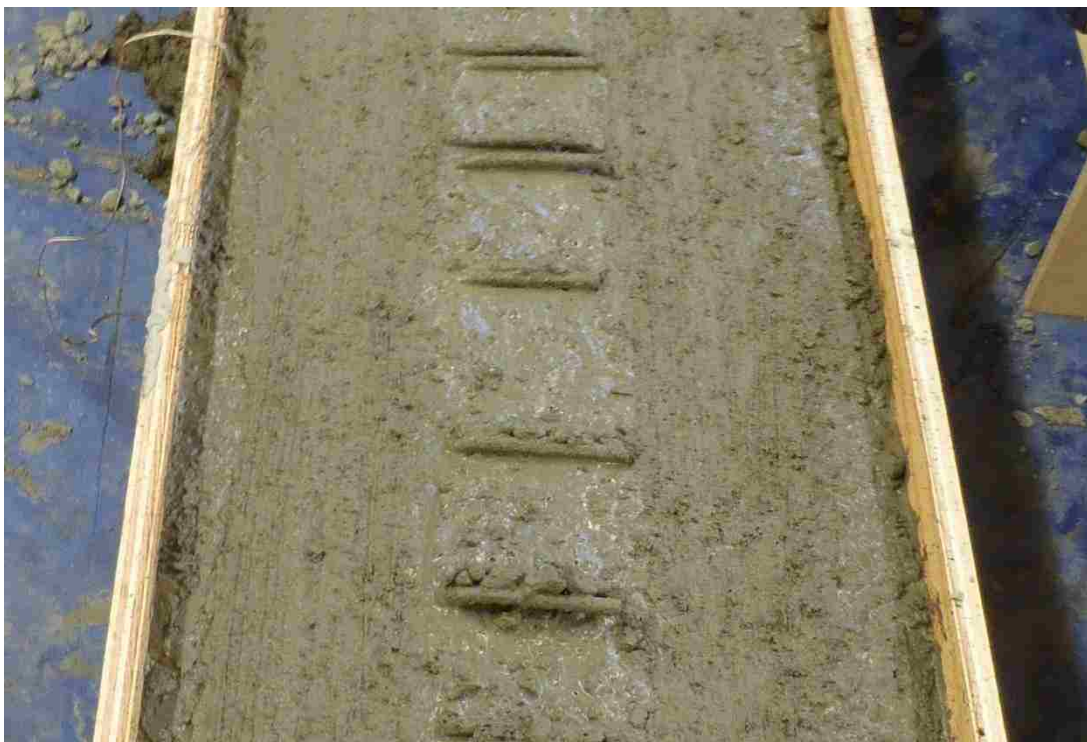
Figure 3.10: The roughened surface of Beam-UF
