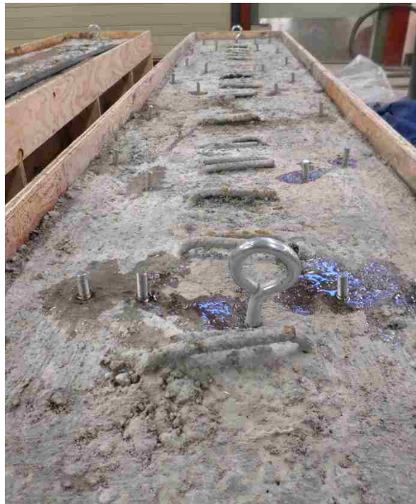
Figure 3.11: Shear dowels installed in top surface of normal concrete in Beam-U
