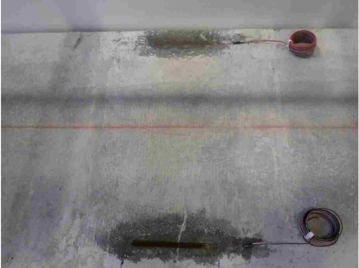
Figure 3.5: Strain gauge installed on top of the concrete
