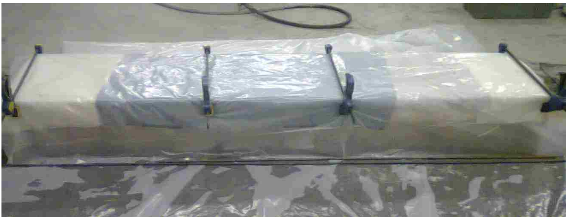
Figure 3.14: Beam-C covered with wet burlap and plastic sheet for curing
