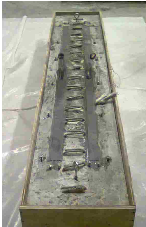
Figure 3.12: CFRP sheets and shear dowels installed in Beam-UF
