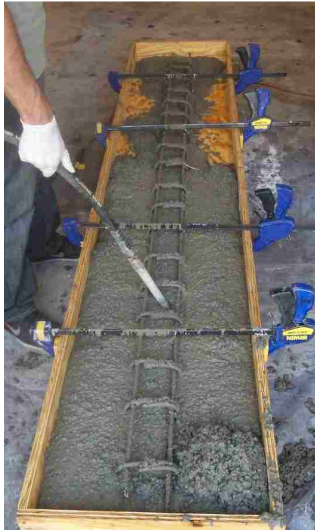
Figure 3.8: Concrete vibrating
