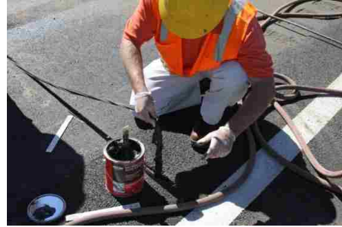
Figure 24. Installation of temperature probes
