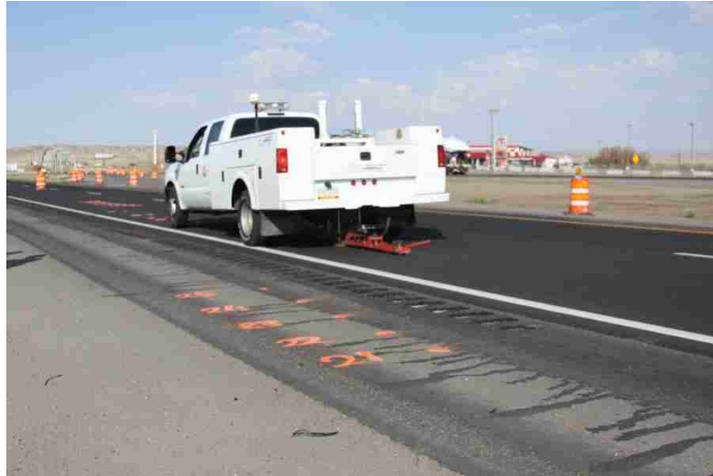
Figure 41. Conduction of FWD test on I-40 pavement
