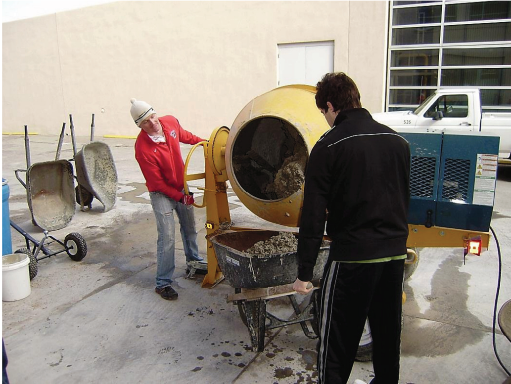
Figure 17: Mixing of concrete, day of casting
