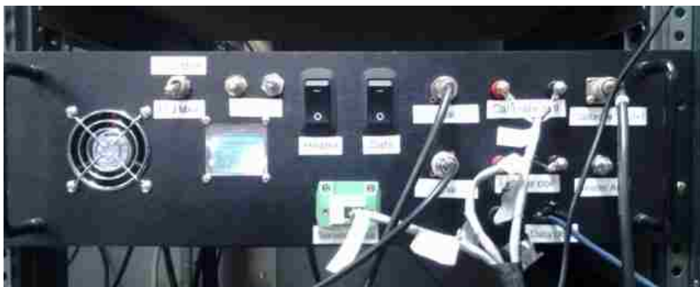
Figure 4.2.10. Calorimeter control panel.
