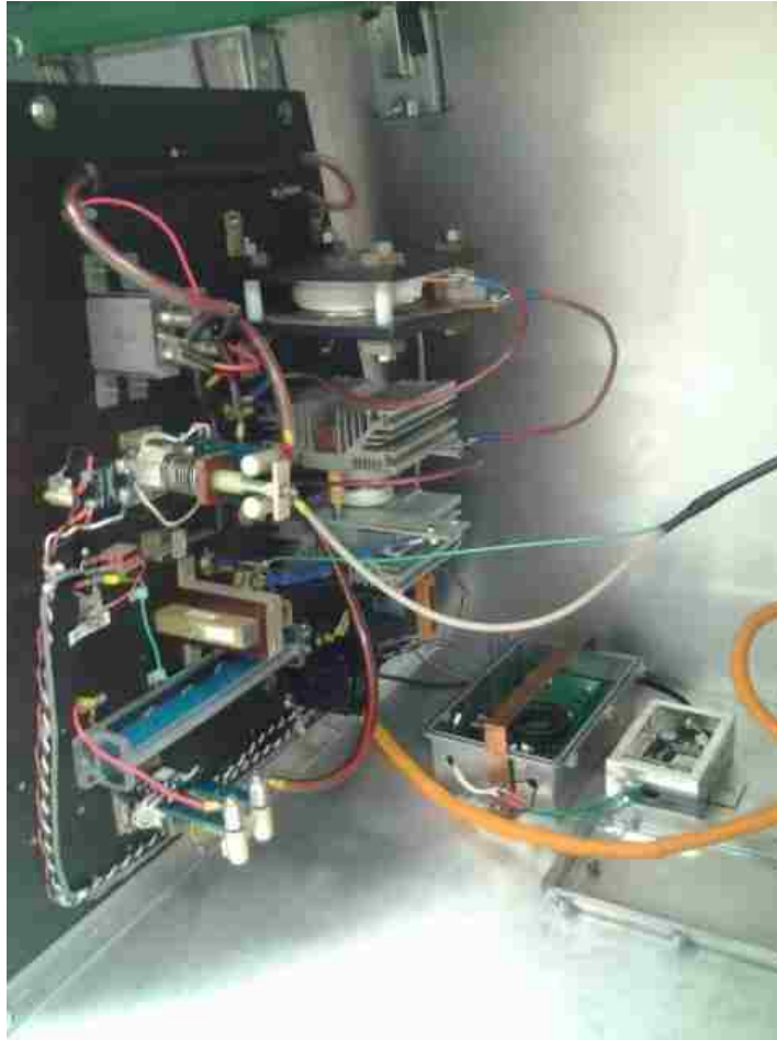
Figure 4.1.4. PULSERAD's pulsed electromagnet circuit.
