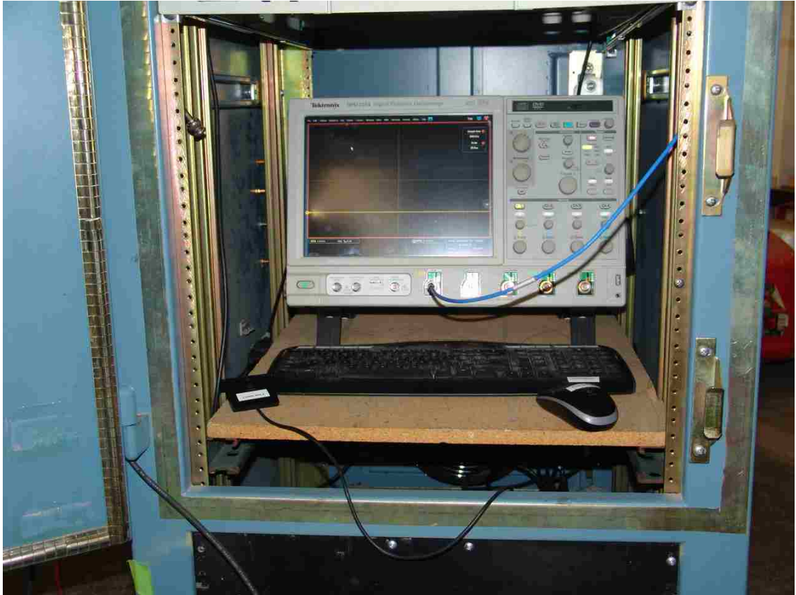
Figure 79. Tek. DPO 7254 Oscilloscope in Screened Enclosure
