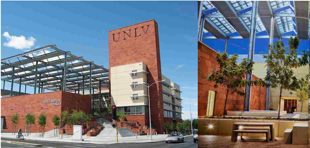
Figure 14. Greenspun Hall, University of Las Vegas is exceptionally arranged to allow for a solar-panel covered courtyard area at the end of a stairway that provides a threshold for interaction and protection from the city streets. The picture on the right shows details that include lighting, landscaping, and site furniture.
