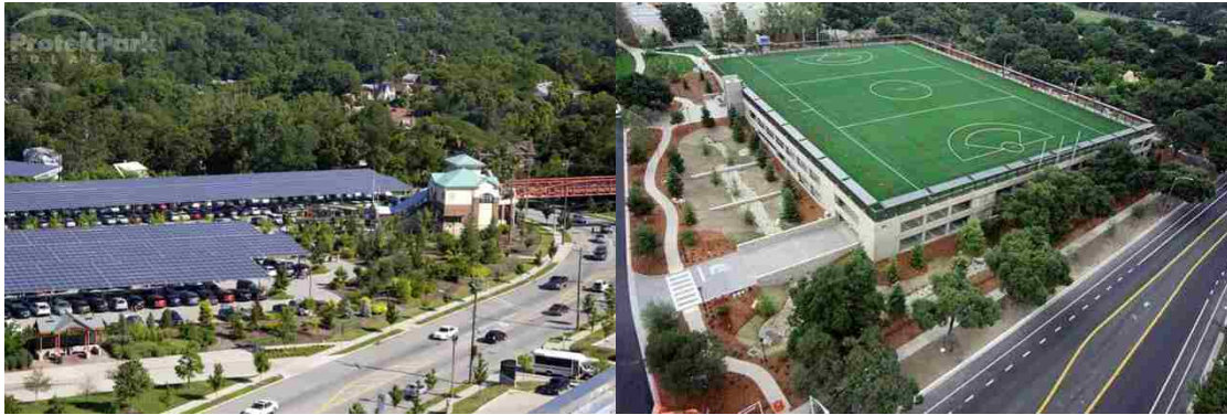
Figure 15. Above (left) is a picture of a solar “parking park” located in Cincinnati, OH. Above (right) is a picture of Pomona College in Claremont, CA which is a three story 600 space parking lot with an athletic field as a roof.
