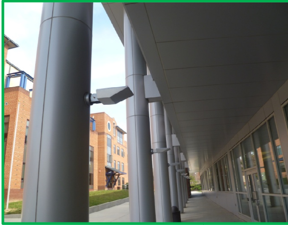
Figure 17: SLCC Exterior. Pillars offer peripheral vision cues with upward facing light fixtures on each pillar along wide walkways.
