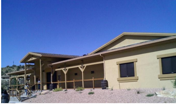
Figure 38. Hualapai Nation Social Services Building. Source: Personal photo.
