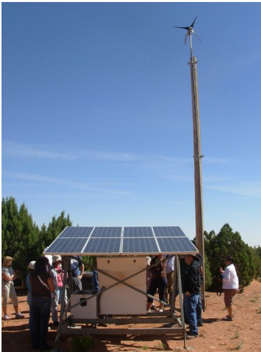
Figure 3. NTUA 880 watt hybrid system in use at Narrow Canyon, Navajo reservation.
