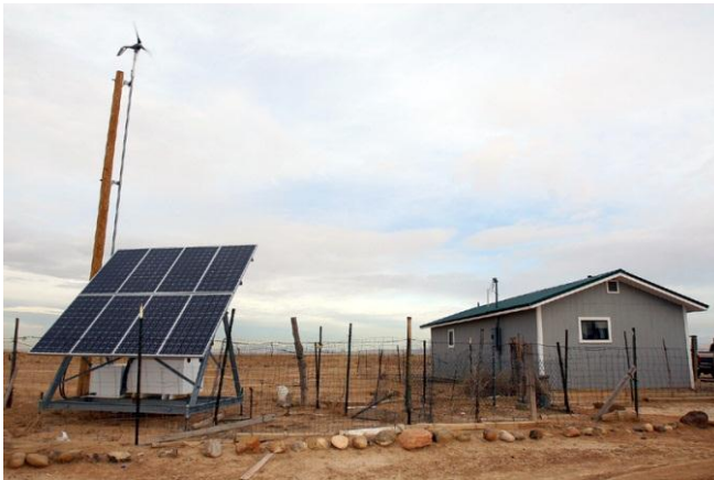
Figure 4. Hybrid system powering rural Navajo home.
