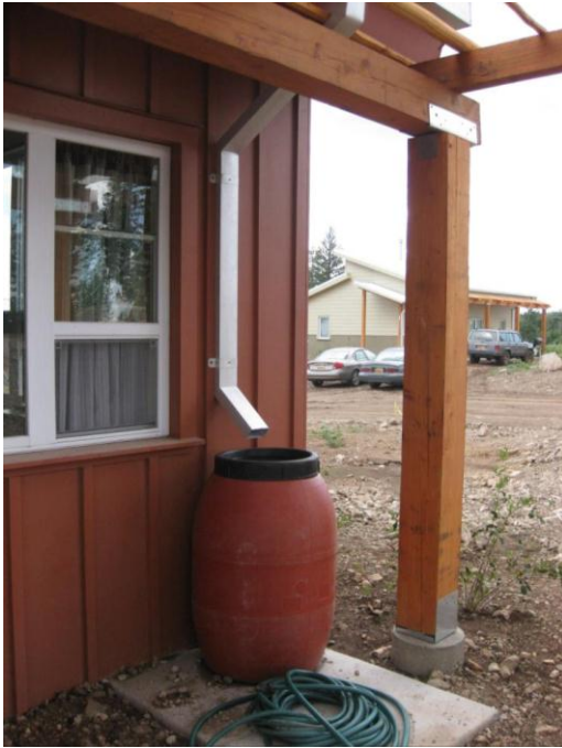
Figure 35. Rain barrels incorporated into new housing at I-Sah'-Din'-Dii.
