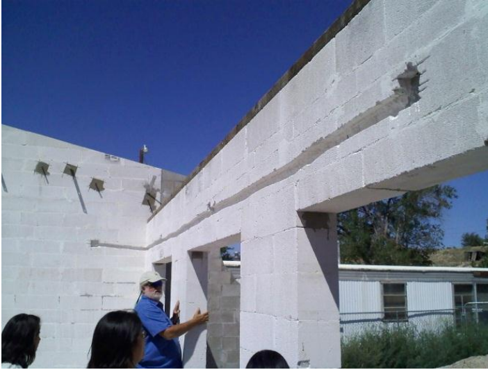
Figure 40. Hualapai Cultural Center: Early construction. Source: Personal photo.
