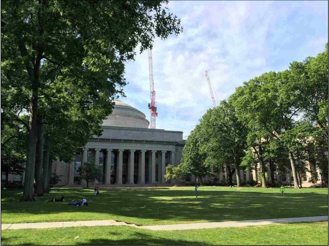
Figure 2. Construction at the Massachusetts Institute of Technology
