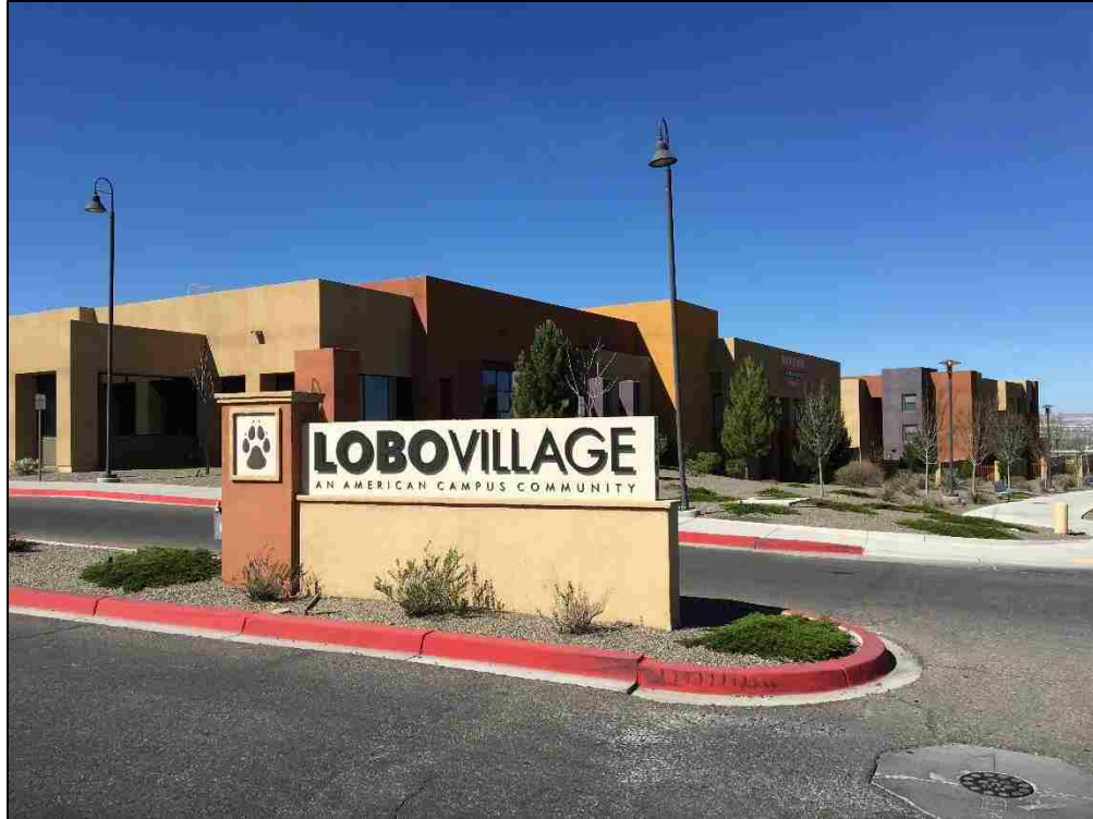
Figure 4. Purpose-Built Student Housing, Albuquerque, NM
