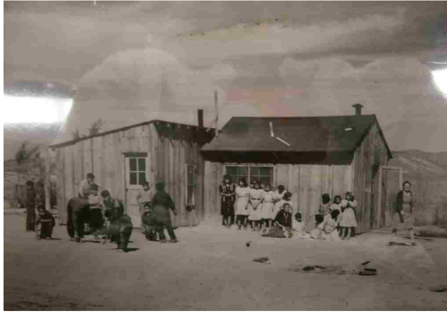
Figure 12. Red Rock Day School dormitory (Photograph No. NE 15-10; “Red Rock Day School, N.M.,” October 7, 1944)
