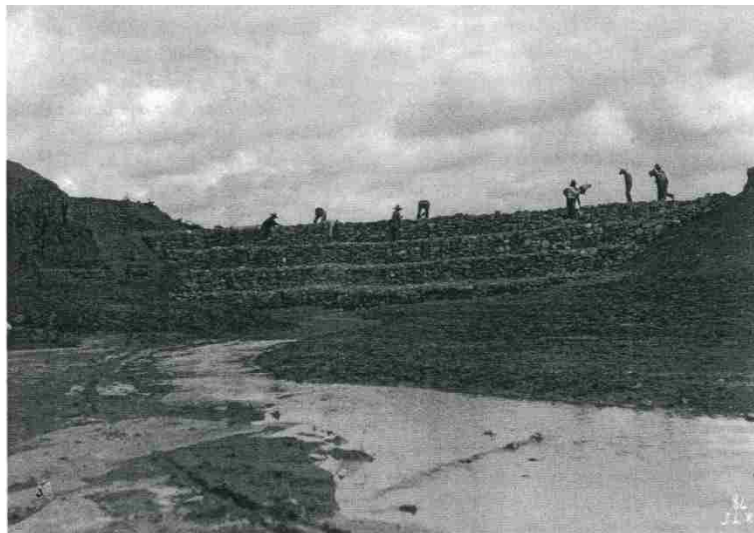
Constructing a dam at Kinlichee.
