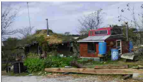
Many homes in Dancing Rabbit, such as this cob house, are built with local natural materials.
