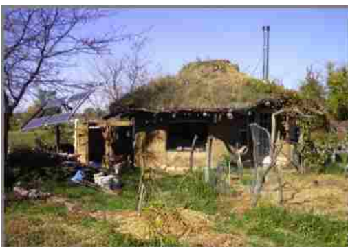
Figure 13: At Dancing Rabbit, structures built with natural materials have excellent thermal mass to control temperatures. Many are also suited with photovoltaic panels.
