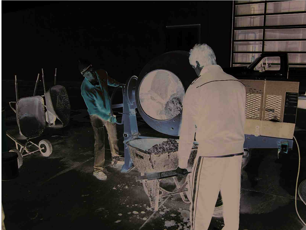
Figure 17: Mixing of concrete, day of casting
