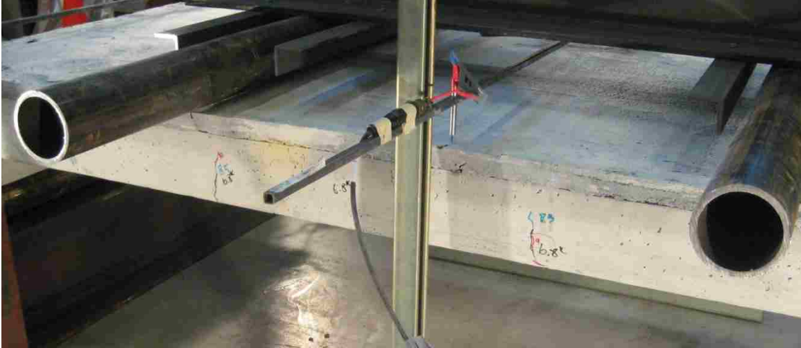
Figure 5.13: Cracking in the strengthened slab at 10 kips (44.5 kN)
