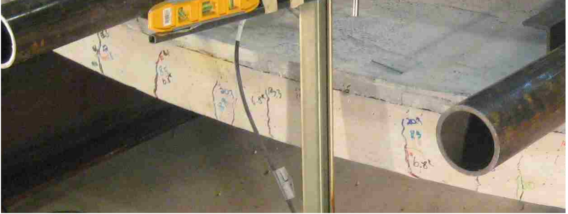
Figure 5.22: UHPC and NVC slab prior to buckling
