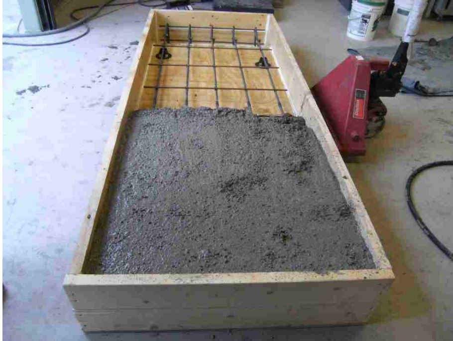
Figure 3.13: Casting the control slab
