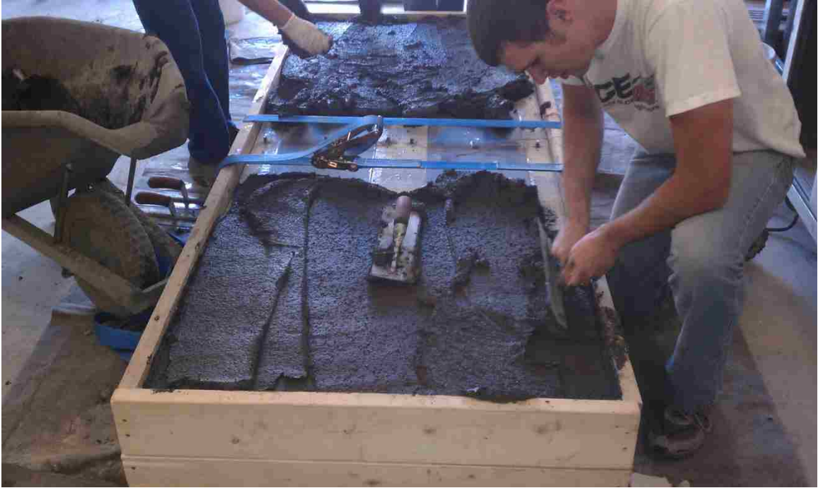
Figure 3.26: Casting the first UHPC batch
