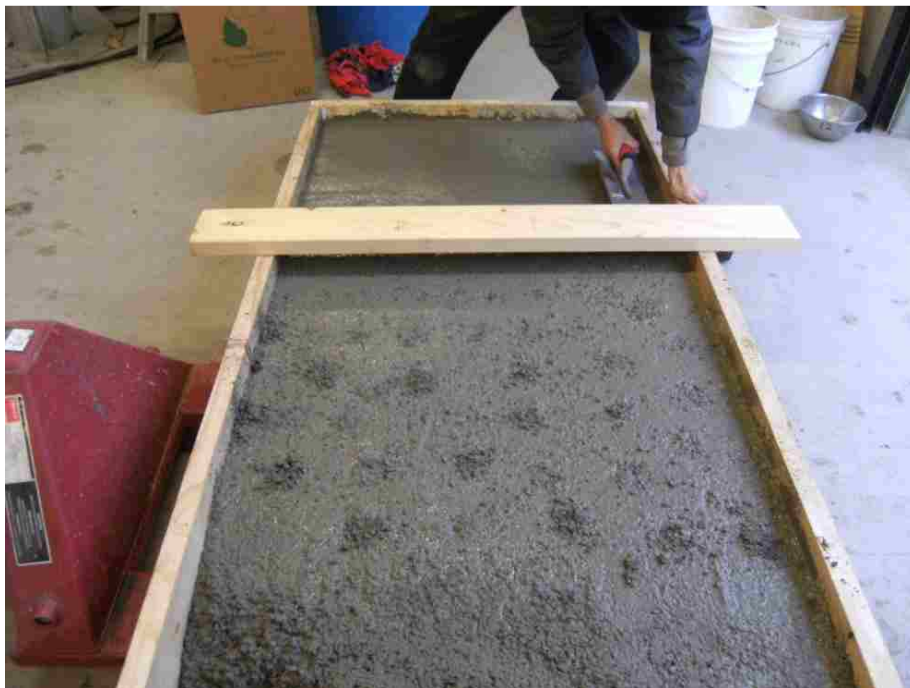
Figure 3.14: Finishing the control slab
