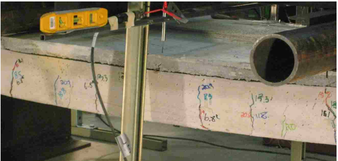
Figure 5.15: Strengthened slab after UHPC debonding
