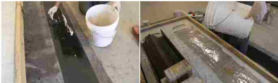
Figure 3.22: Application of the epoxy to the CFRP and slab
