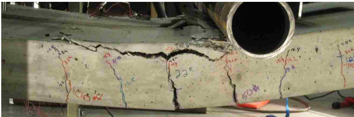
Figure 5.3: Failure due to concrete crushing in the control slab
