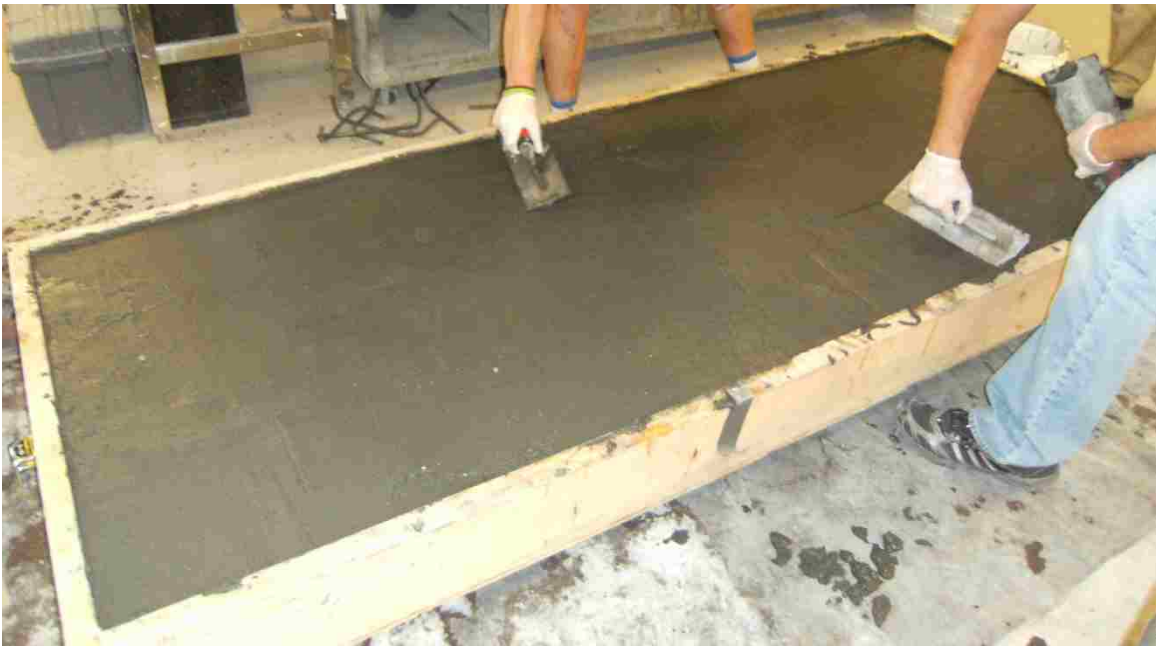
Figure 3.27: Finishing the second UHPC batch
