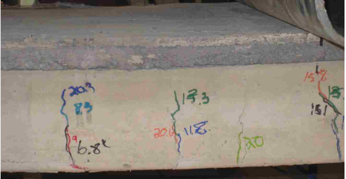
Figure 5.14: Strengthened slab prior to UHPC debonding
