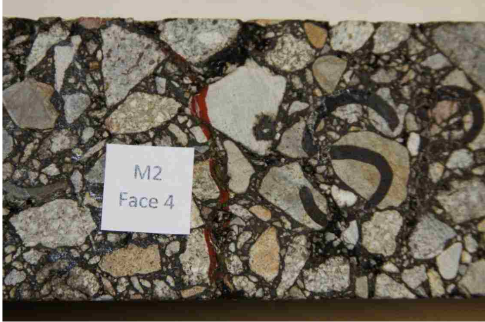
Figure 6.8 Fatigue Cracking in HMA Beam Sample SP-III-M2
