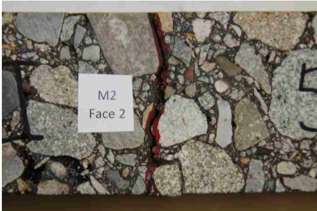
Figure 6.3 Fatigue Cracking in HMA Beam Sample SP-II-M2
