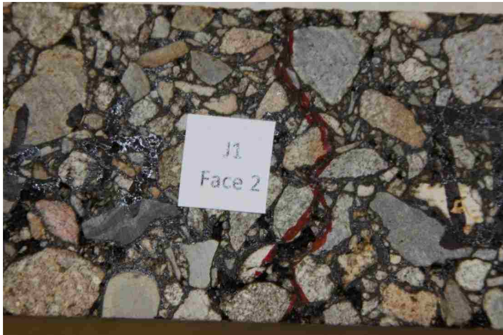
Figure 6.7 Fatigue Cracking in HMA Beam Sample SP-III-J1
