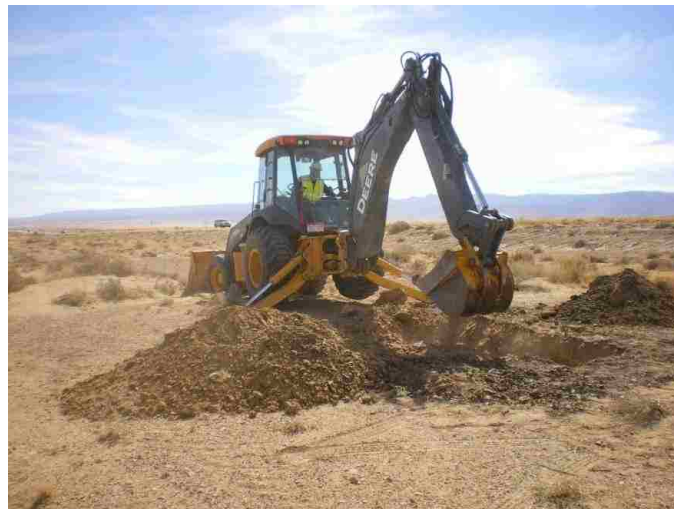
Figure 3.2 Backhoe Loader Removing Soil Used In This Study
