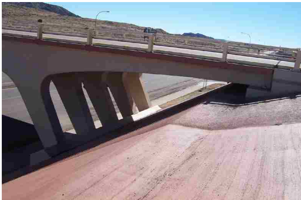
Figure 5-2 K-Frames of Bridge 7937.
