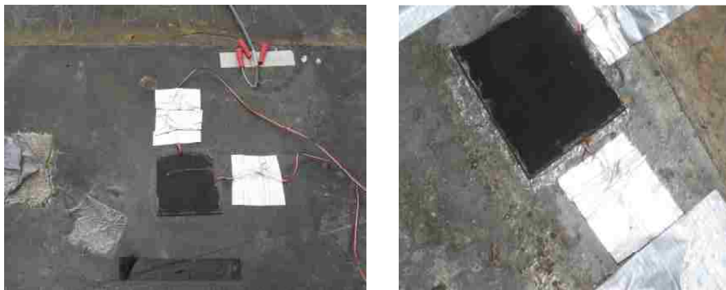
Figure 5-53 Covered strain gauges attached to the FRP sheets.
