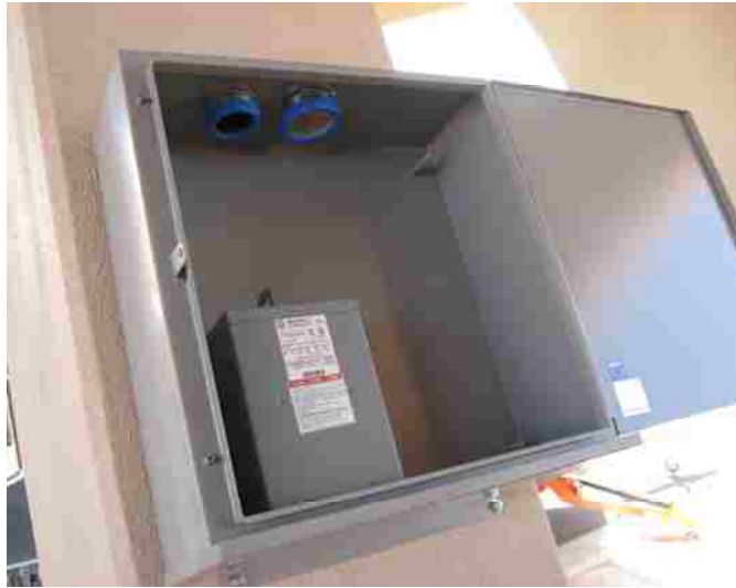
Figure 5-47 Steel box used for housing the data acquisition system and all SHM components.
