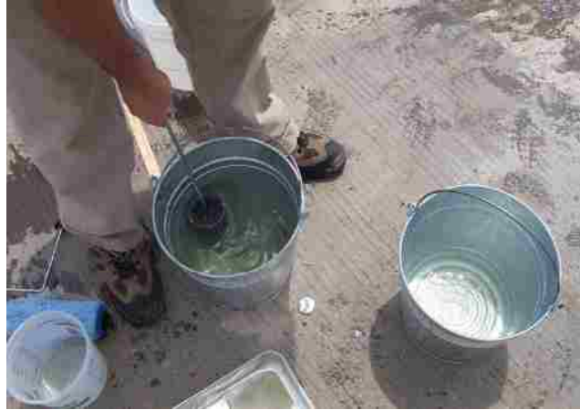
Figure 5-14 Mixing resin and hardener according to specific mixing ratio.
