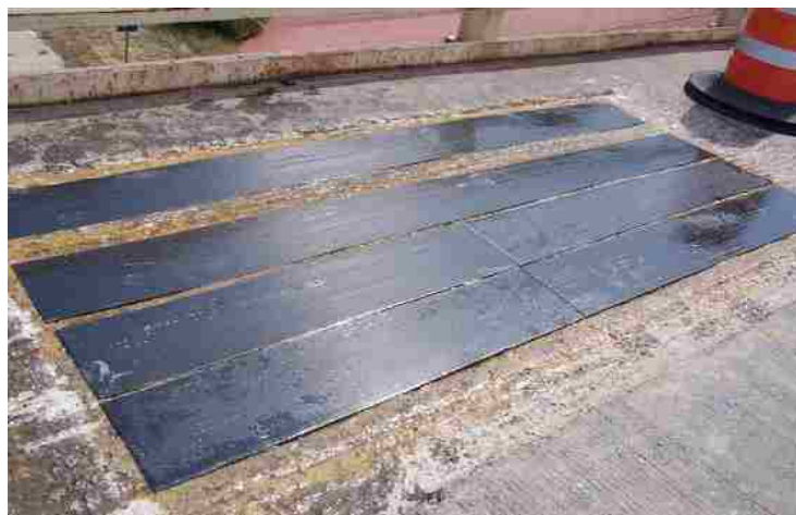
Figure 5-15 FRP strips attached to the concrete surface.
