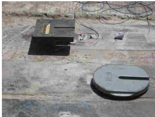
Figure 5-52 Weights applied on top of each installed strain gauge.
