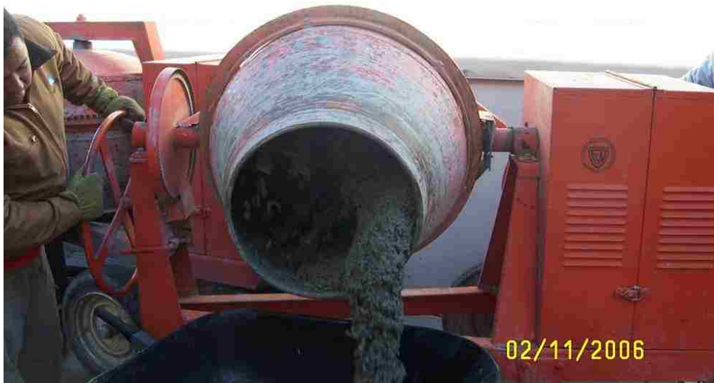
Figure 3.2. Mixing of fresh concrete
