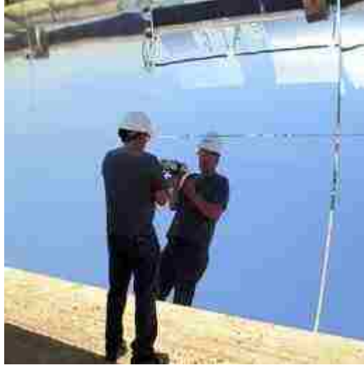
Figure 1.8: ReflecTech ® Installed in the Field [5]
