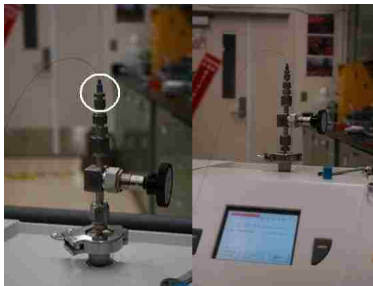
Figure 6 A Nanoport fitting is plumbed to quadrupole mass spectrometer for He leak test.
