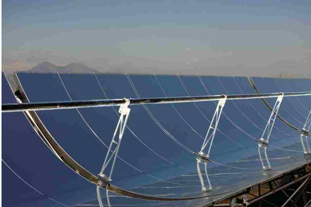
Figure 1. Concentrating solar trough system. Copyright and credit: SkyFuel 2009. Used by permission. Location, Albuquerque, NM (US Department of Energy 2012).
