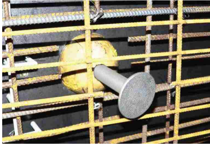
Figure 11: Rebar reinforced concrete form with lifting pin. Photo provided by a lifting pin system retailer Patterson-online.com is not necessarily the rebar structure in the anchors, but represents an assumed likely interior. (Lifting Pin Anchor System 2011)
