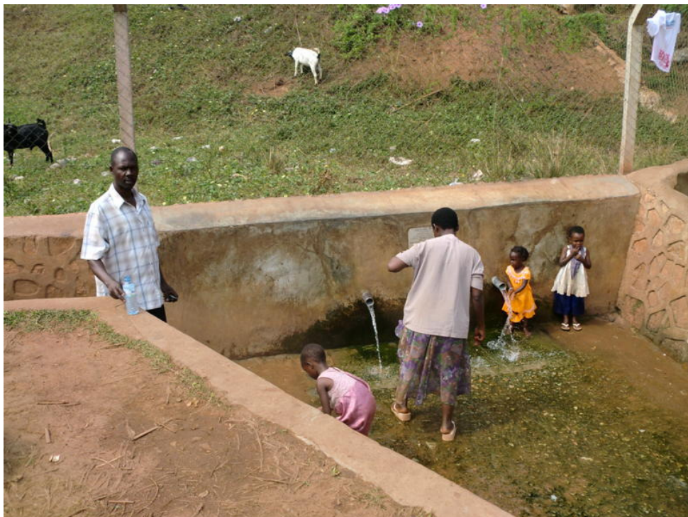
Fig 6.1: Example of a spring inside the town of Kampala, the capital of Uganda. Spring water is used for drinking, cooking and bathing. Please note the concrete slab and the fencing behind the spring in order to try to protect the intake area
