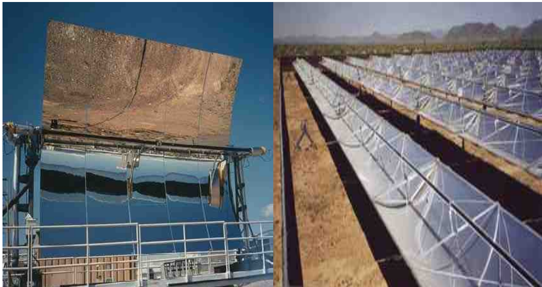
Figure 2.6c Parabolic trough collectors.
