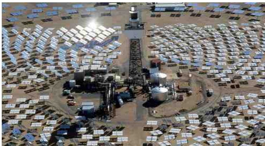
Figure 2.6a A Central Receiver System [13].
