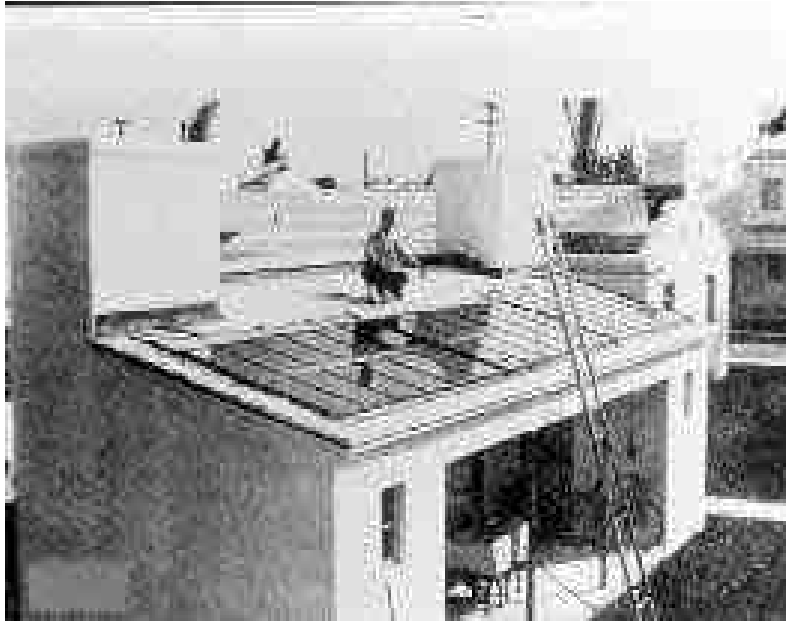
Figure 2.1b Solar water collector with separated storage tank [6].
