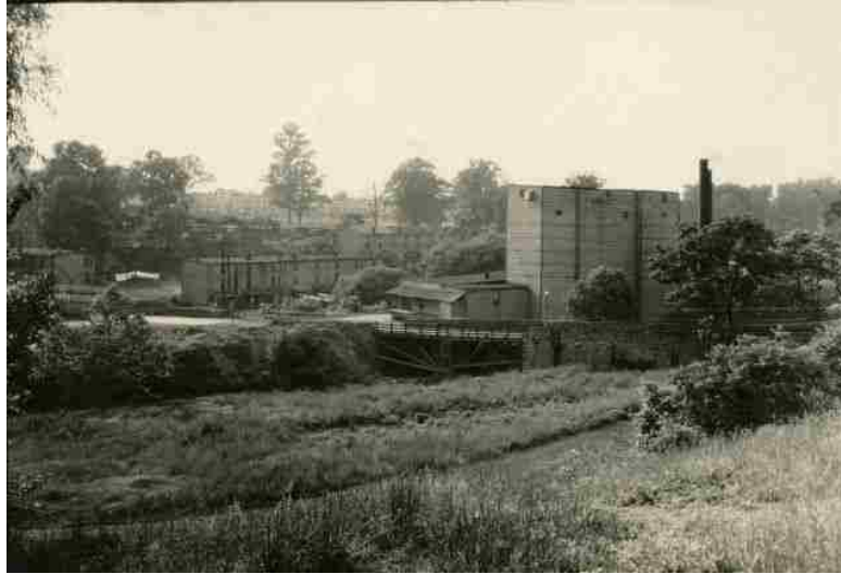
Figure 55. Industrial buildings along the Delaware County side of Cobbs Creek, 1912. (City Parks Association).
