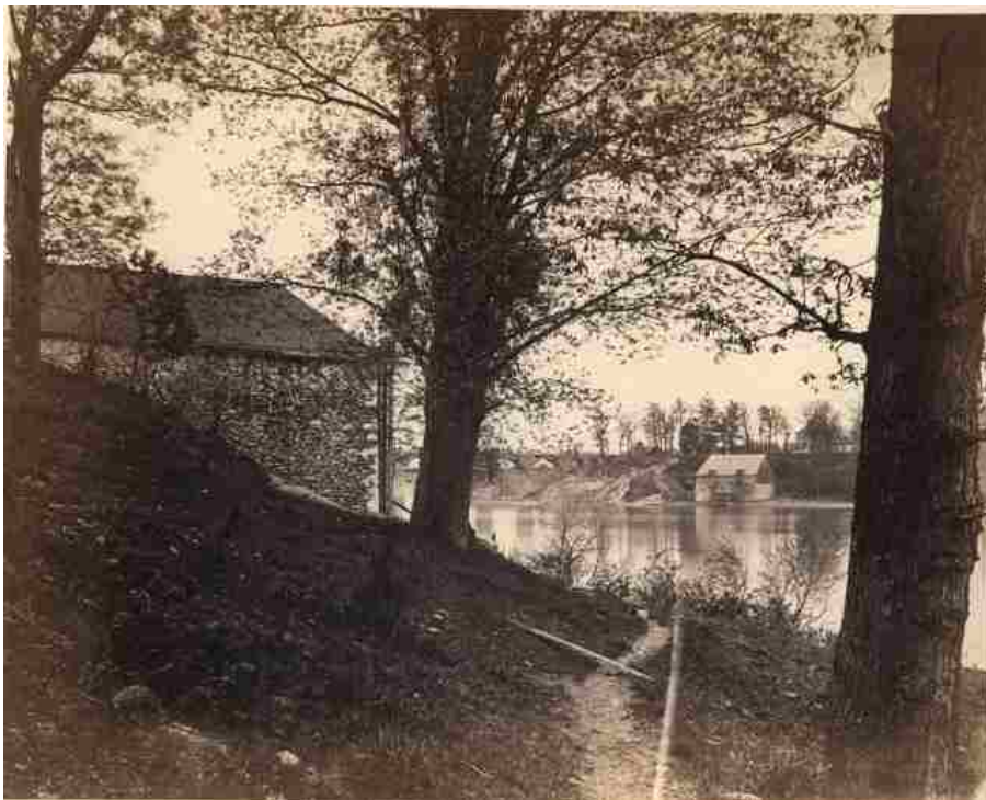
Figure 16. Large ice houses, used by the lager beer industry, line both banks of the Schuylkill, c. 1860s. Prior to the improvements of the original plan, these buildings needed to be demolished (Fairmount Park Historic Resource Archive).
