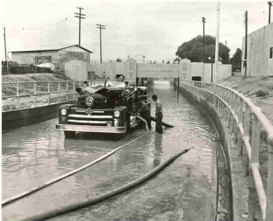
Figure 17. A fire-engine crew pumping water out of the Bonanza underpass, date unknown. (image courtesy of UNLV Special Collections)
