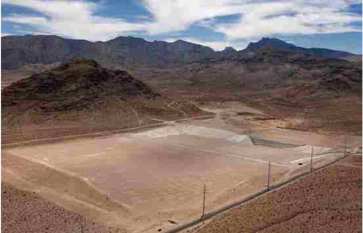
Figure 10. Ann Road Detention Basin, northeast of Las Vegas. (image courtesy of CCRFCD)
