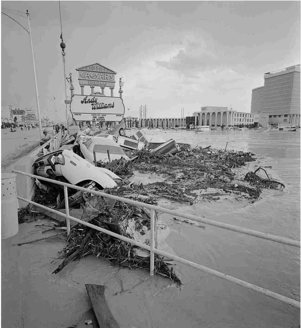
Figure 24. July 3, 1975 Clark County Public Works situated a crane on the Strip to remove cars.
