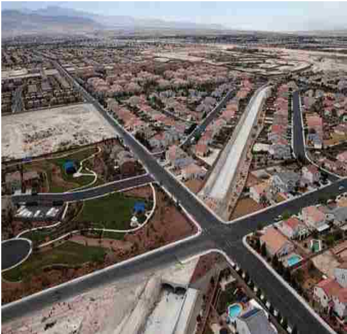
Figure 29 Las Vegas Middle Branch Channel (image courtesy of CCRFCD)
