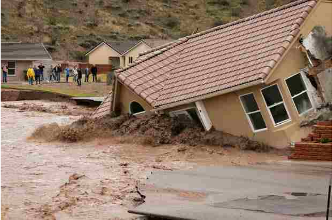
Figure 35. A home washing into the Virgin River in the Beaver Dam, Arizona. (photo credit given to Associated Press)
