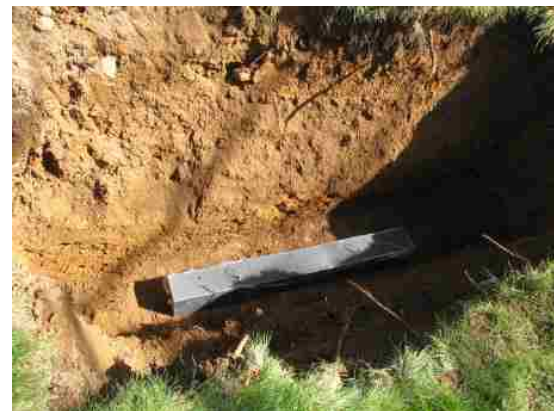
(c) Installed sensors in the box with temperature probes before burying
