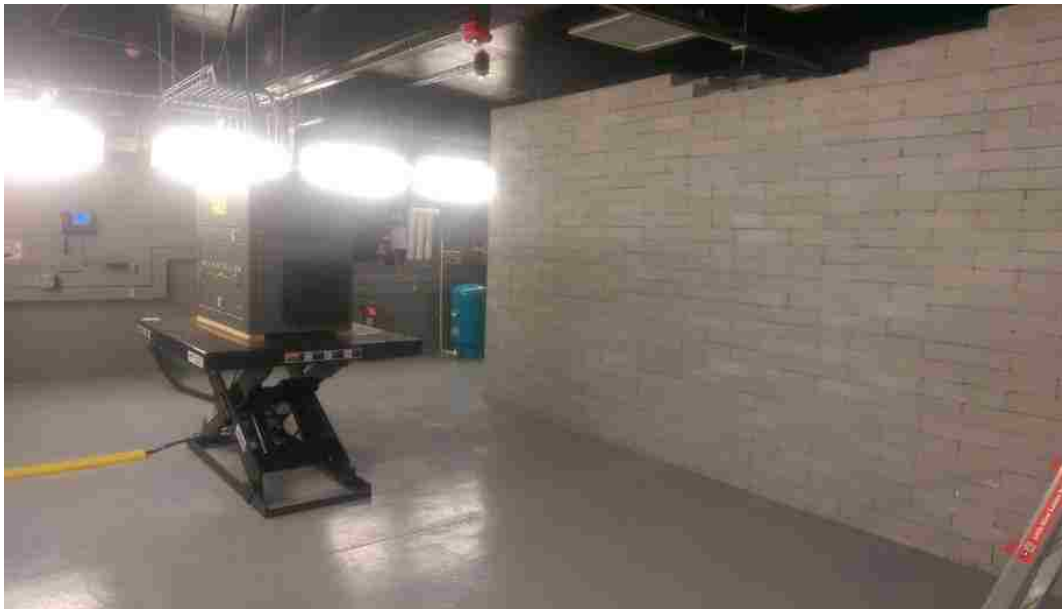
Figure 10. Varian M6 inside accelerator facility
