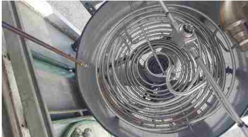
Figure 14. Air Cooled Heat Rejection Heat Exchanger
