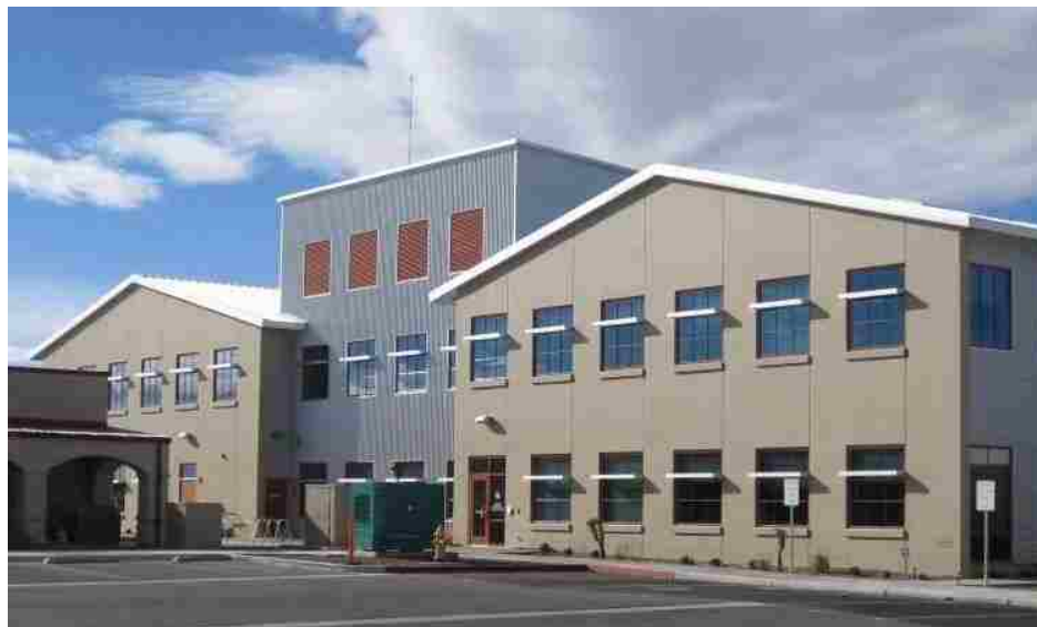
Figure 12. LCROGB East-Facing Metal and Concrete Exterior Walls.
