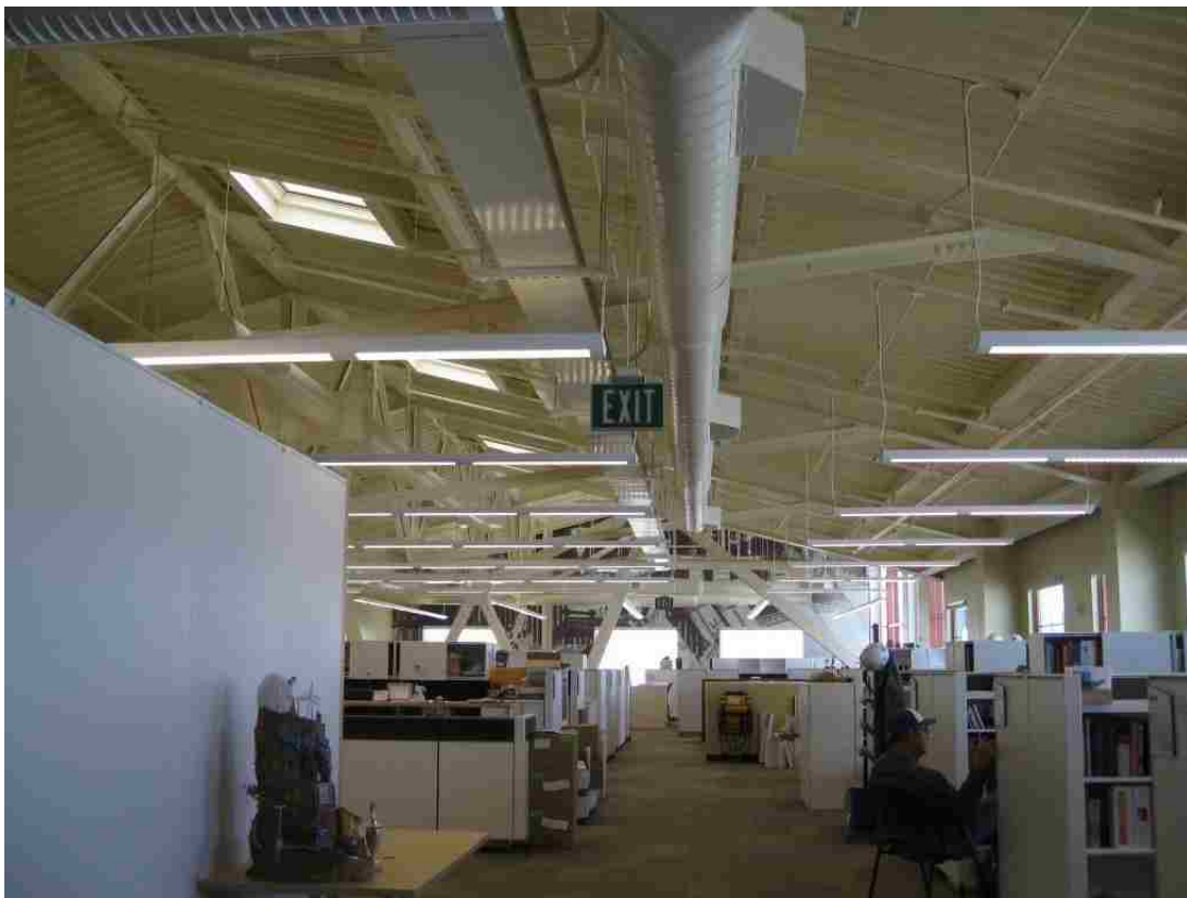
Figure 4. LCROGB Interior View of Second Floor.
