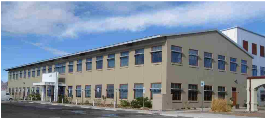
Figure 14. LCROGB South- and East-Facing Walls With Window Light Shelves.
