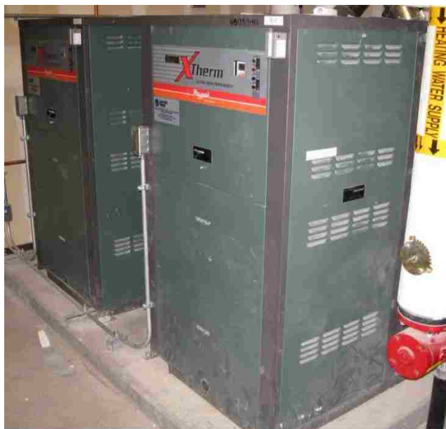
Figure 36. Raypak XTherm Boilers.
