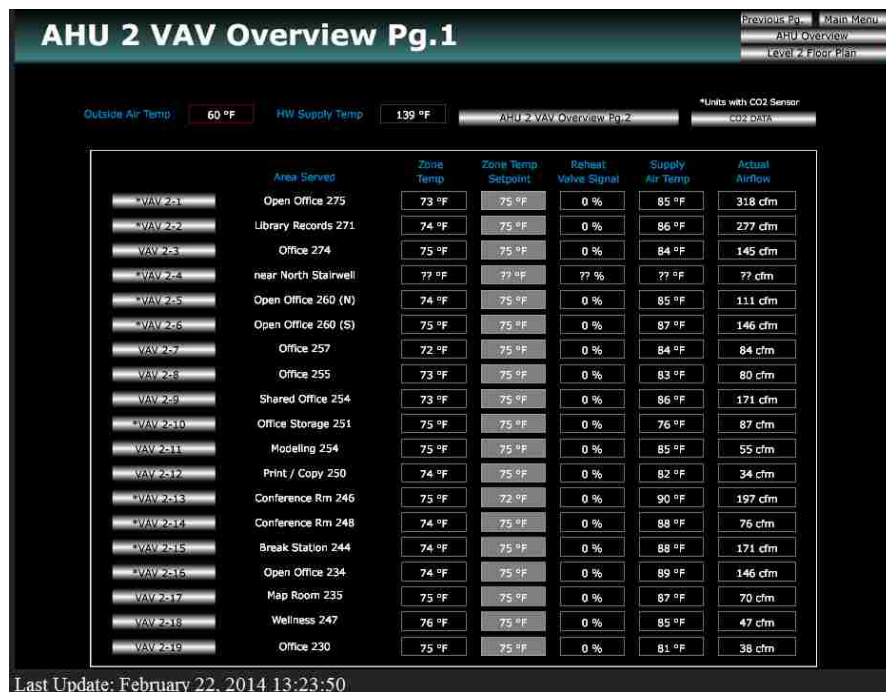
Figure 41. BMS Variable Air Volume Overview Sample Page.
