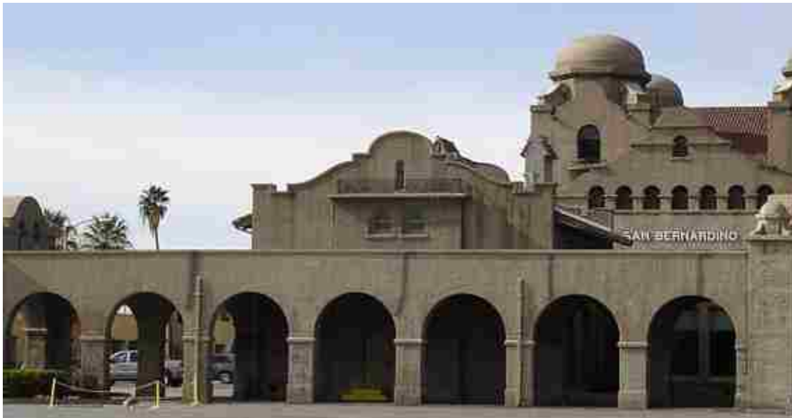
Figure 6. Modern view of the Santa Fe depot in San Bernardino. Though typically described as an example of “Moorish Revival” architecture, the distinction between this and Mission Revival may be more of an attempt to distance the building and the railroad company from associations with Mexico. During 1917-1918 when the building was constructed, Mexico was in the midst of violent and protracted revolution. Additionally, an effort by Germany to arrange a military alliance between itself and Mexico came to light in 1917. The initiative included an offer to assist Mexico in reclaiming territory lost in the Mexican-American War, specifically Arizona, New Mexico and Texas. (Photo by the author, January 2010).
