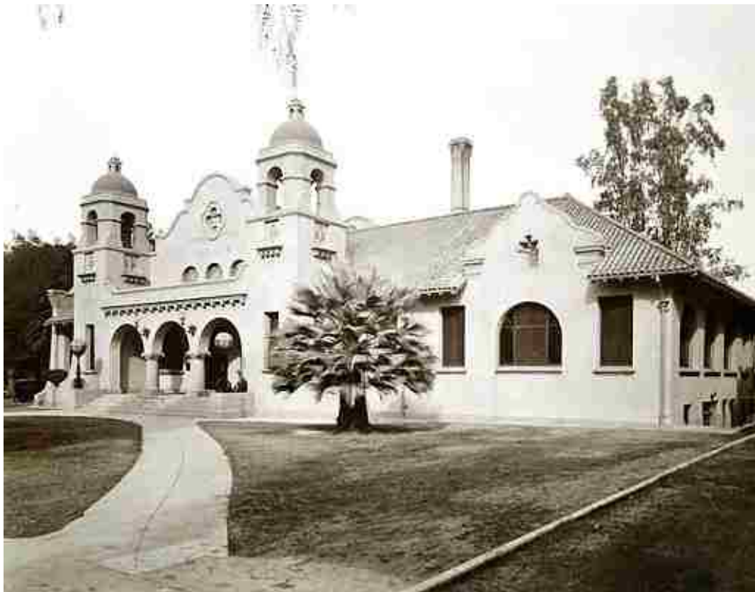
Figure 9. Riverside’s Carnegie Library (1903-1964), designed by Arthur Benton, exemplified the architectural motifs characteristic of the Mission Revival style. The design is fundamentally ecclesiastical, presumably to suggest that the library was a temple of learning. This metaphor was one that Andrew Carnegie specifically encouraged in libraries he funded. The steps leading to the entrance (visible on the left) symbolized personal elevation, and the lamps alongside the steps represented enlightenment. (Riverside Public Library, Photo LIB RIV CEN CAR V 22 CLD2-98)
