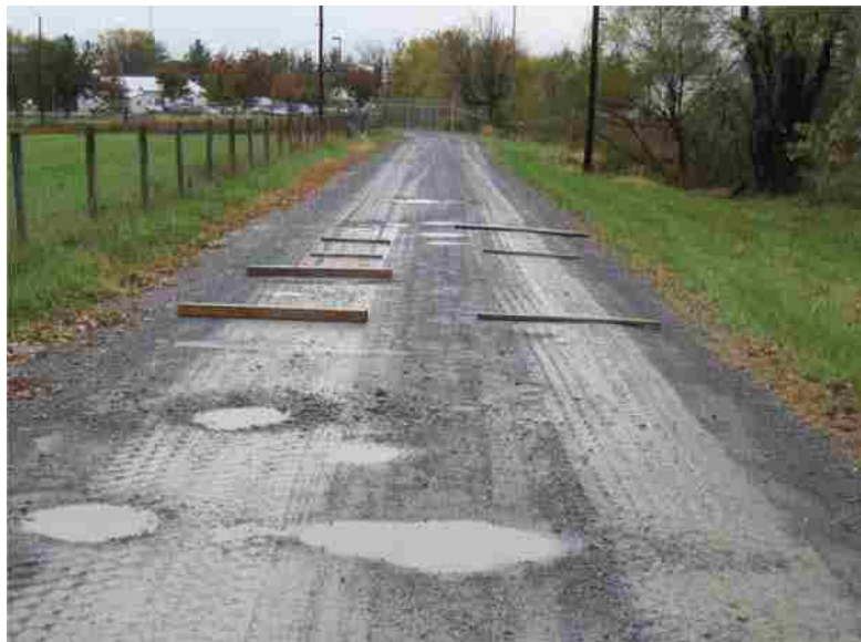
Figure 4.11 MRAP Road Course
