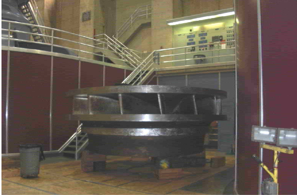
Figure 36: Turbine Runner being staged for further modifications and repairs [2].
