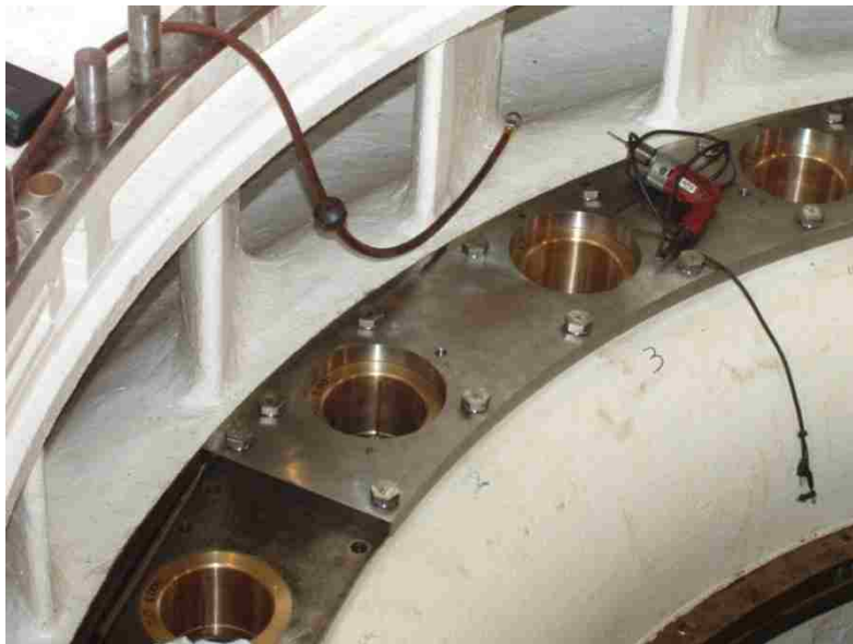
Figure 11: New wear plates bolted below wicket gates [2].
