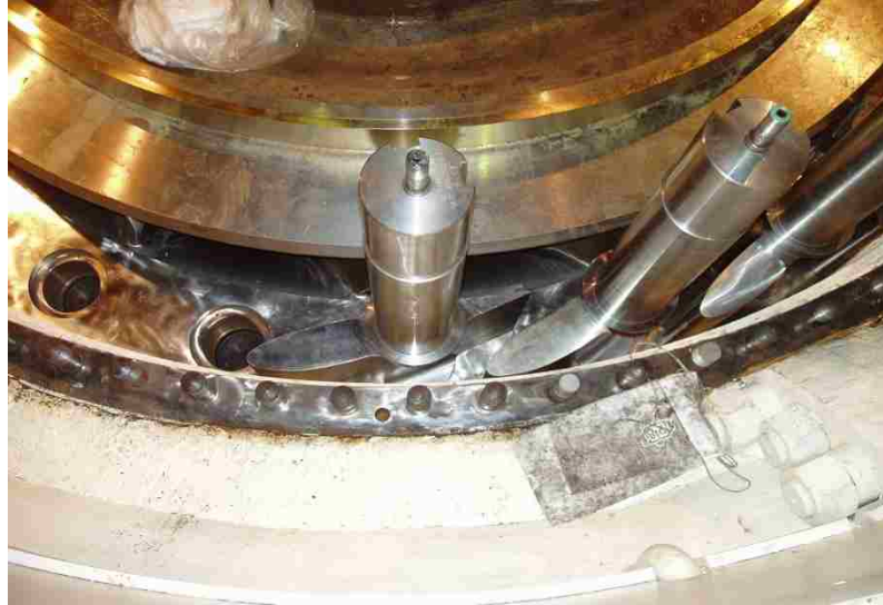
Figure 16: New Wicket Gates being installed [2].
