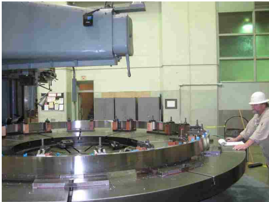
Figure 19: Machining the turbine runner seal rings on the Cincinnati [2].
