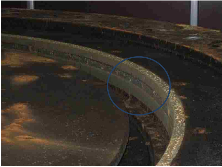
Figure 18: Lower Seal Ring [2].
