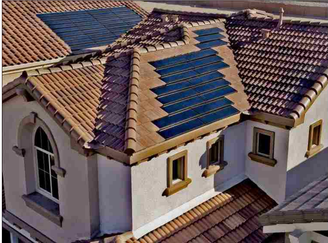
FIGURE 3 - ROOF TILE PV CELLS AT VILLA TRIESTE
