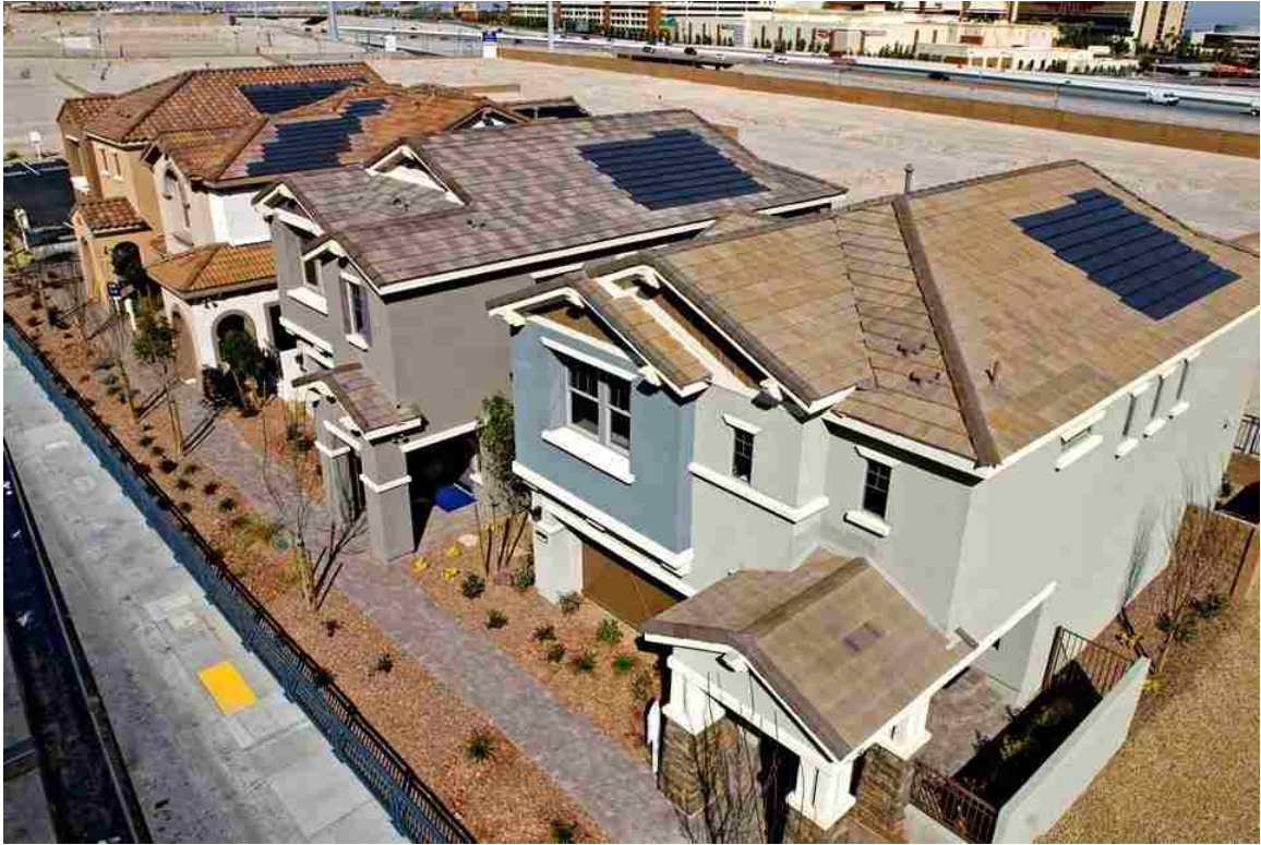
FIGURE 10 - PV PANELS ON EACH VILLA TRIESTE MODEL HOME
