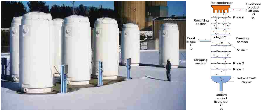
Figure 2.2: (left) A standard distillation assembly to capture Kr and Xe. (Right) A description of one column of the distillation assembly.[18]
