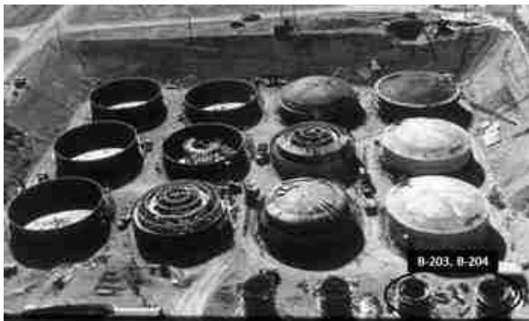
Figure 1.2. Left: construction of 12 waste tanks at the Hanford site. Right: diagram of a single-shell tank.
