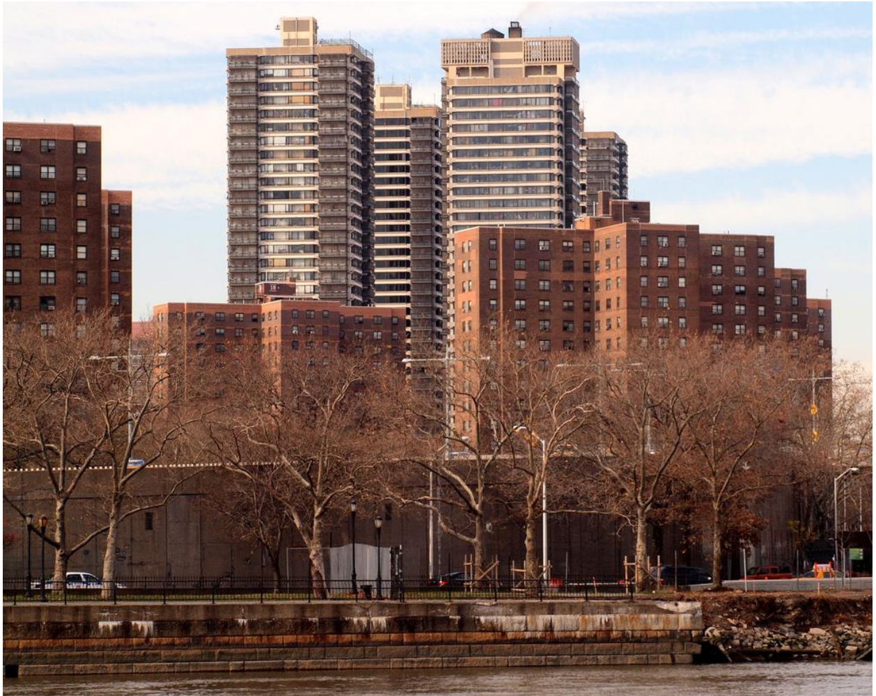
Figure A.2 Taino Towers
