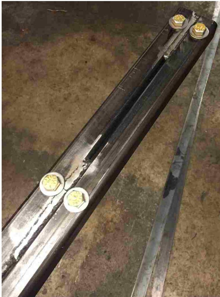
Figure 48. Welded support beam.
