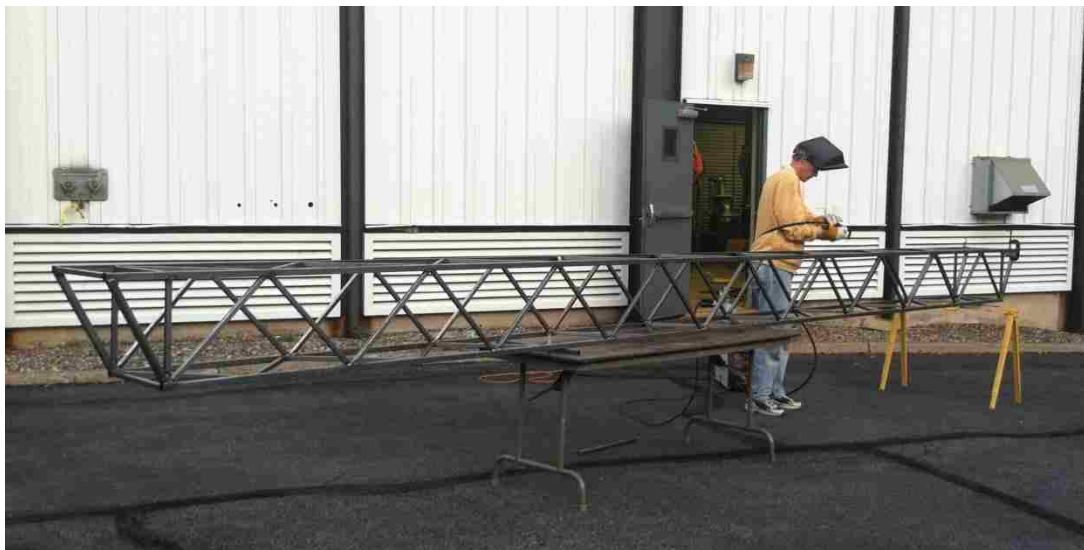
Figure 36: Finish Welding Support Truss
