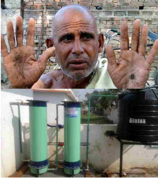
Figure 3.17. (A) A resident of Ballia, UP suffering from arsenicosis lesions on his hands before the installation of the arsenic treatment system (top); (B) the installed, simple HAIX-NanoFe system, which produced over 1 million liters of arsenic-safe water since opening.
