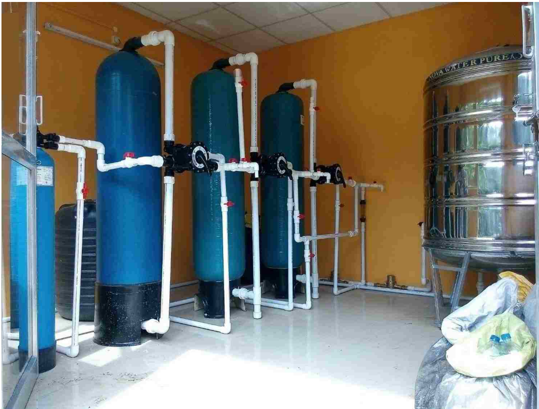
Figure 3.12. Baduria arsenic treatment system with three treatment columns (SAC-Fe, HAIX-NanoZr, and WAC-Na) and one activated carbon post-treatment column. (R-L: Influent→I→ II→III→IV). Black chemical dosing tanks (200 L) for Column I (ferric chloride) and Column III (sodium carbonate) can be seen behind the respective tanks. The stainless steel treated water storage tank can be seen on the right.
