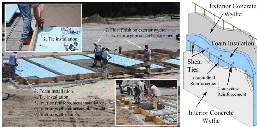
Figure 1: Insulated wall panel construction and configuration
