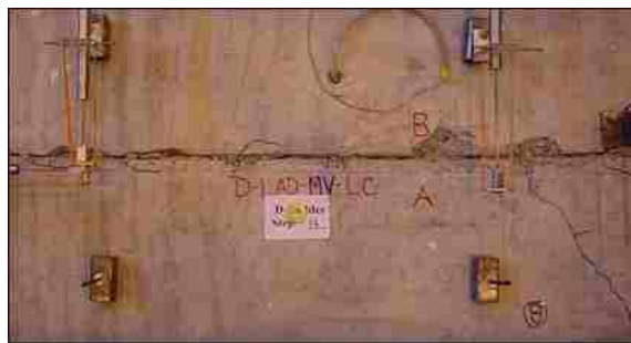
Figure 4.24. Damage state at 0.33-in shear opening
