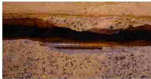
Figure 4.13. Damage state at 2.0-in tensile opening
