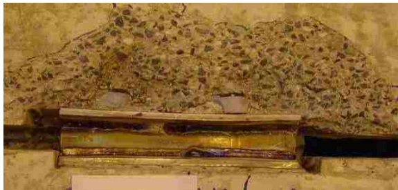
Figure 4.38. Damage state at 0.75-in shear opening
