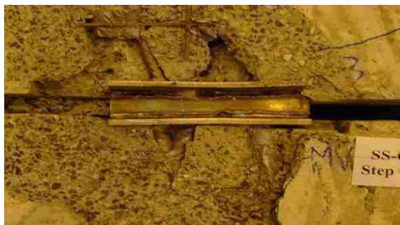
Figure 4.39. Damage state at 4.5-in shear opening
