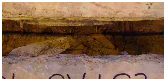
Figure 4.30. Damage state at 1.08-in shear opening
