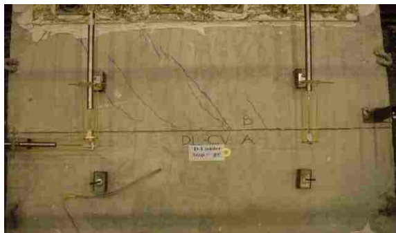
Figure 4.25. Damage state at 0.59-in shear opening
