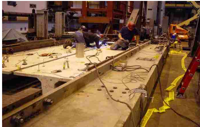
Figure 7.2. Field welding of connections between panels
