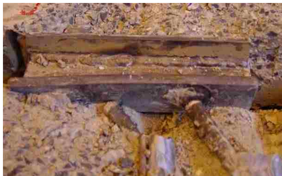
Figure 4.35. Damage state at 3.5-in shear opening
