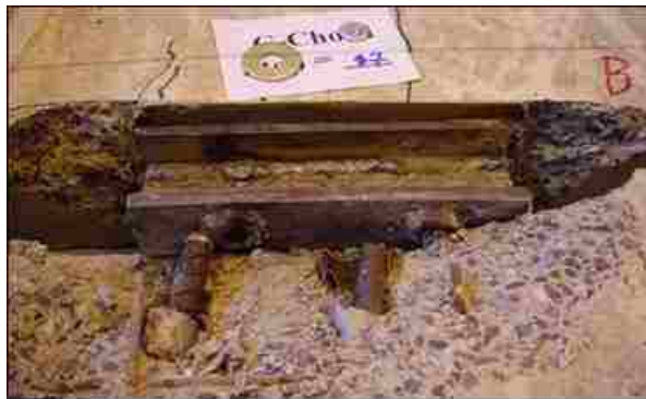
Figure 4.36. Damage state at 1.98-in shear opening
