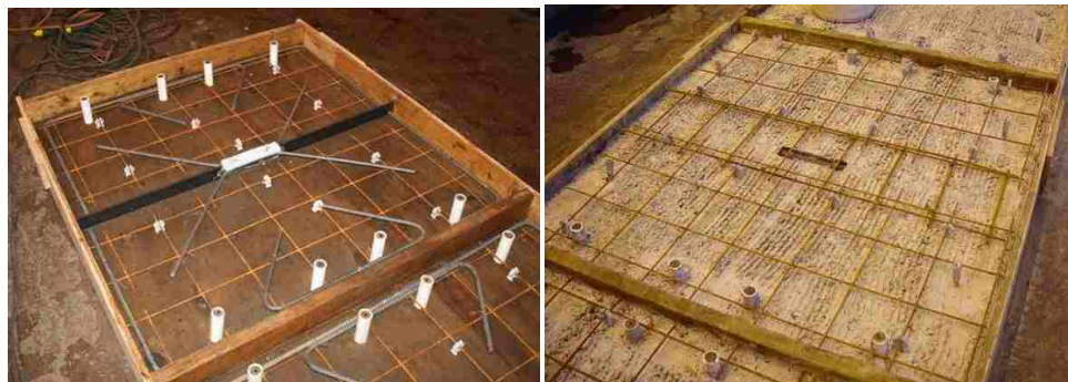
Figure 4.4. Ductile ladder with hairpin connector
