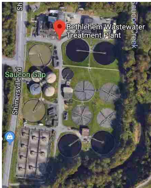
Figure 3-1. Satellite view of the Bethlehem WWTP in Bethlehem, PA (40°37'03.5"N 75°20'00.2"W). 82
