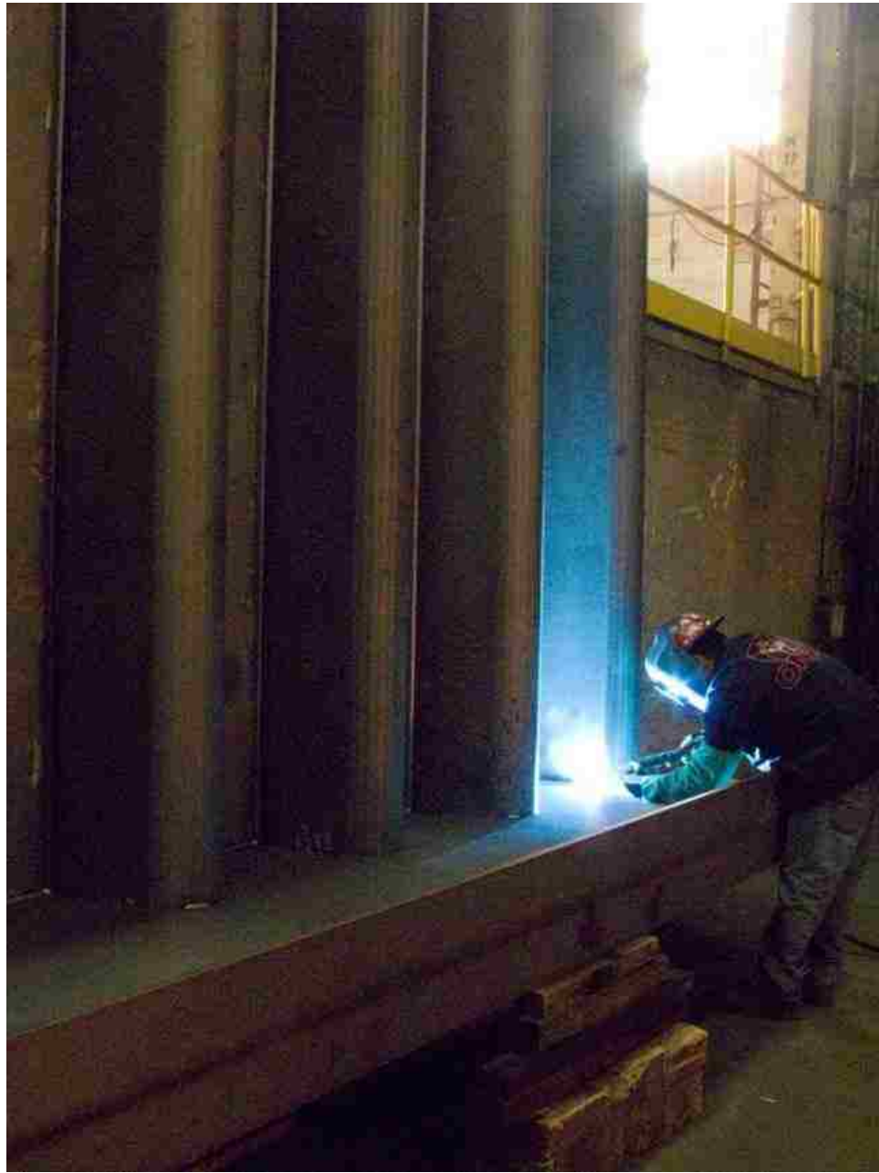
Figure 101 Rib-to-floor beam welding in 2F position
