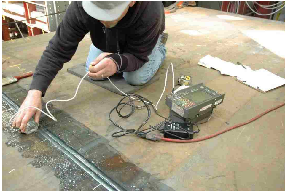
Figure 119 UT of CJP Deck Splice
