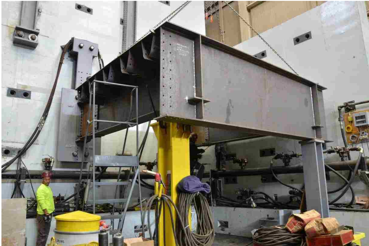
Figure 105 Installation of the east panel
