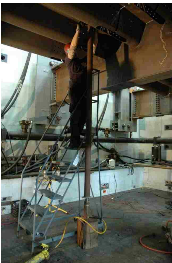
Figure 110 Jacking of west panel
