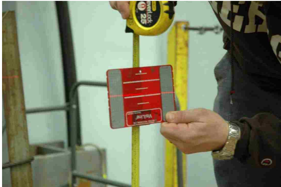
Figure 120 Deck level measurements using laser
