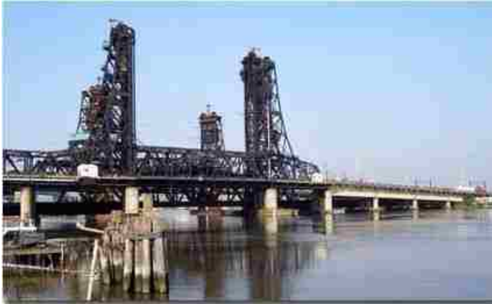
Figure 1 The lift bridge
