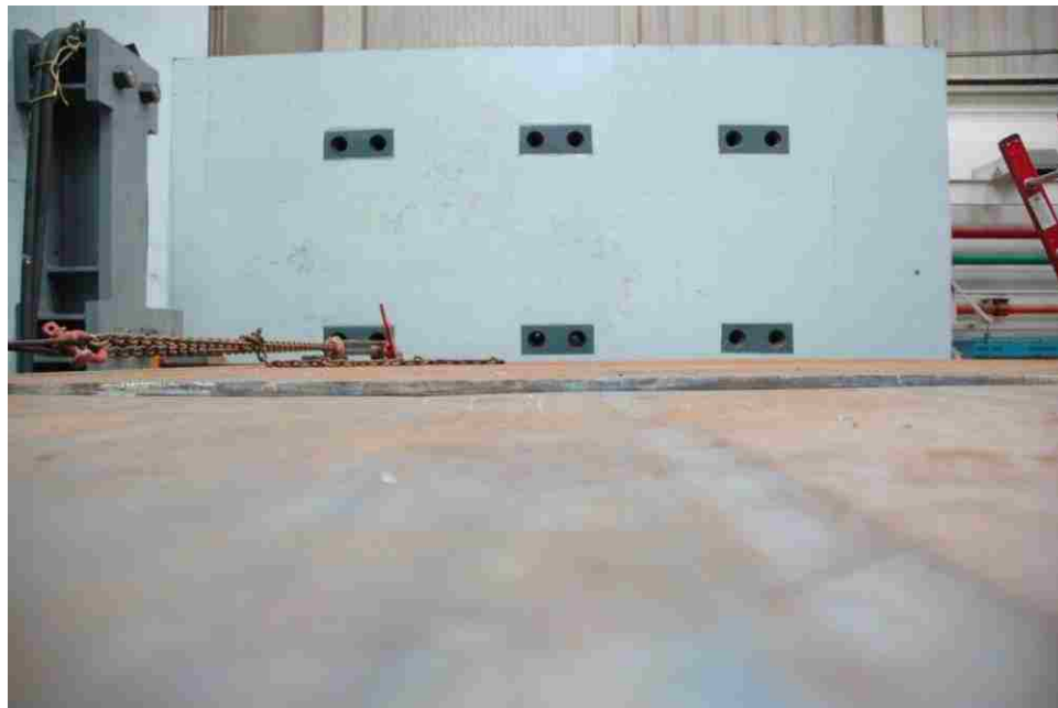
Figure 108 Elevation difference at splice location before tacking
