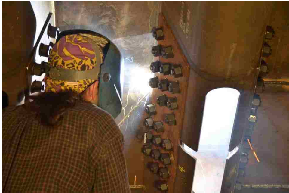
Figure 115 Back gouge and re-welding in between the ribs
