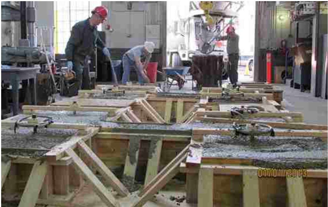
Figure 3-46: Concrete casting of test specimens
