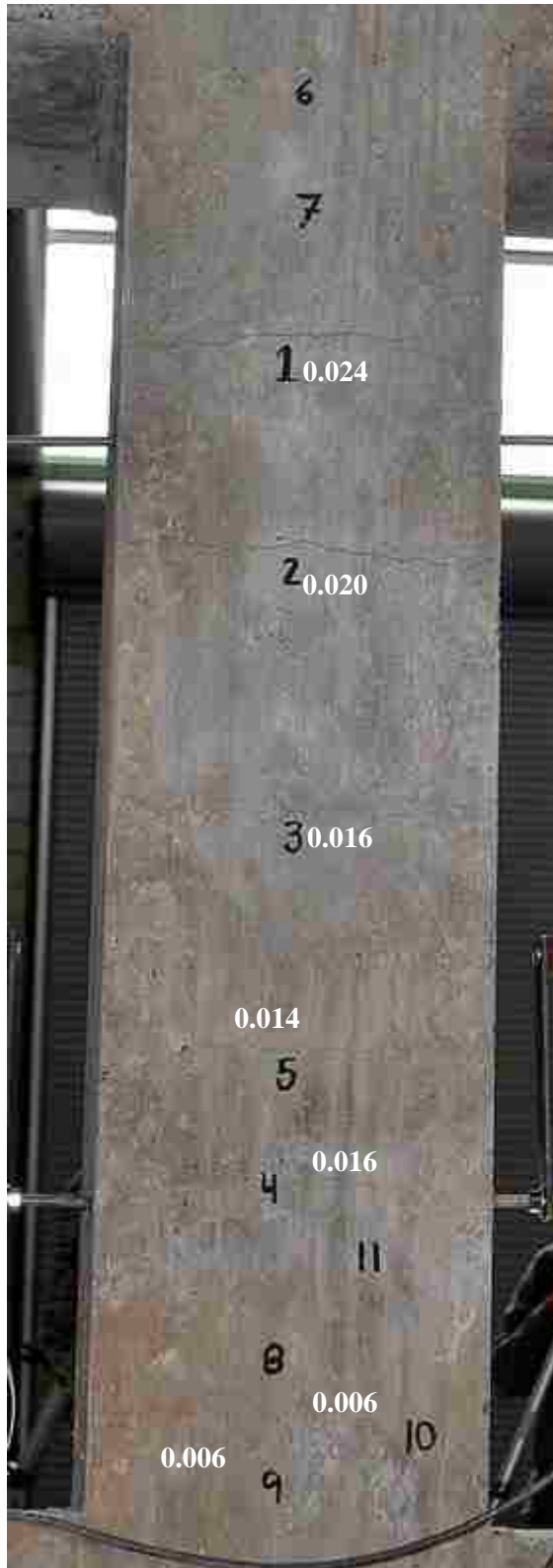
Figure 4-85: Cracks on east face of TS01 at Load Step 19
