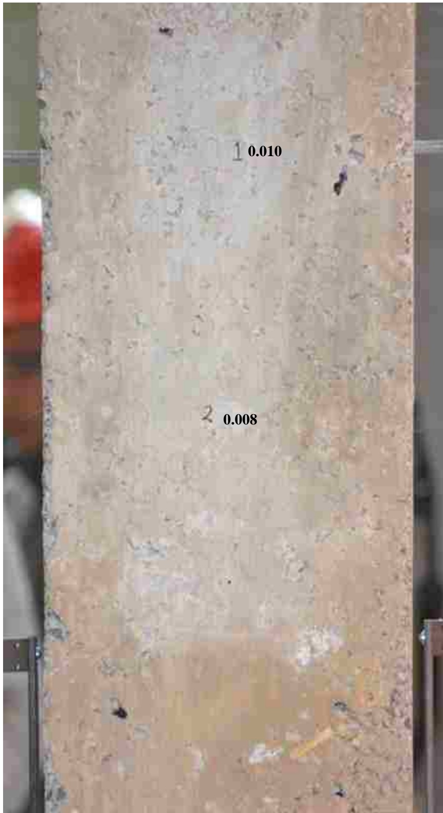
Figure 4-91: Cracks on east face of TS02 at Load Step 08
