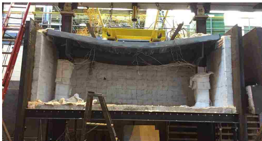
Figure 71 – Unprotected Beam after Failure
