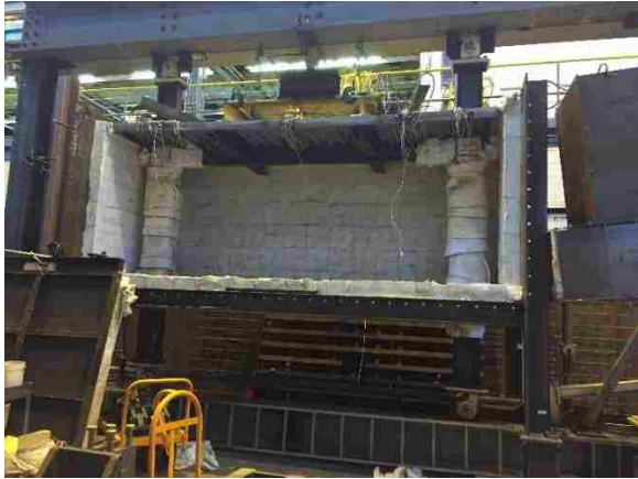
Figure 6 – Protective Ceramic Blankets on Columns and Beam Connections
